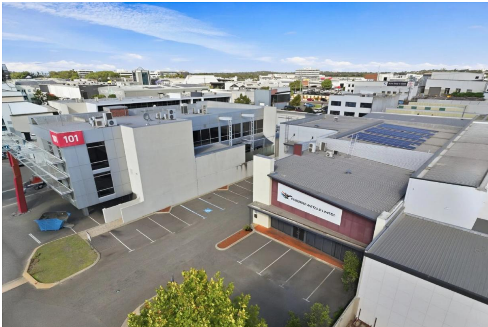
The Australian Demonstration Plant property, Osborne Park, Perth
