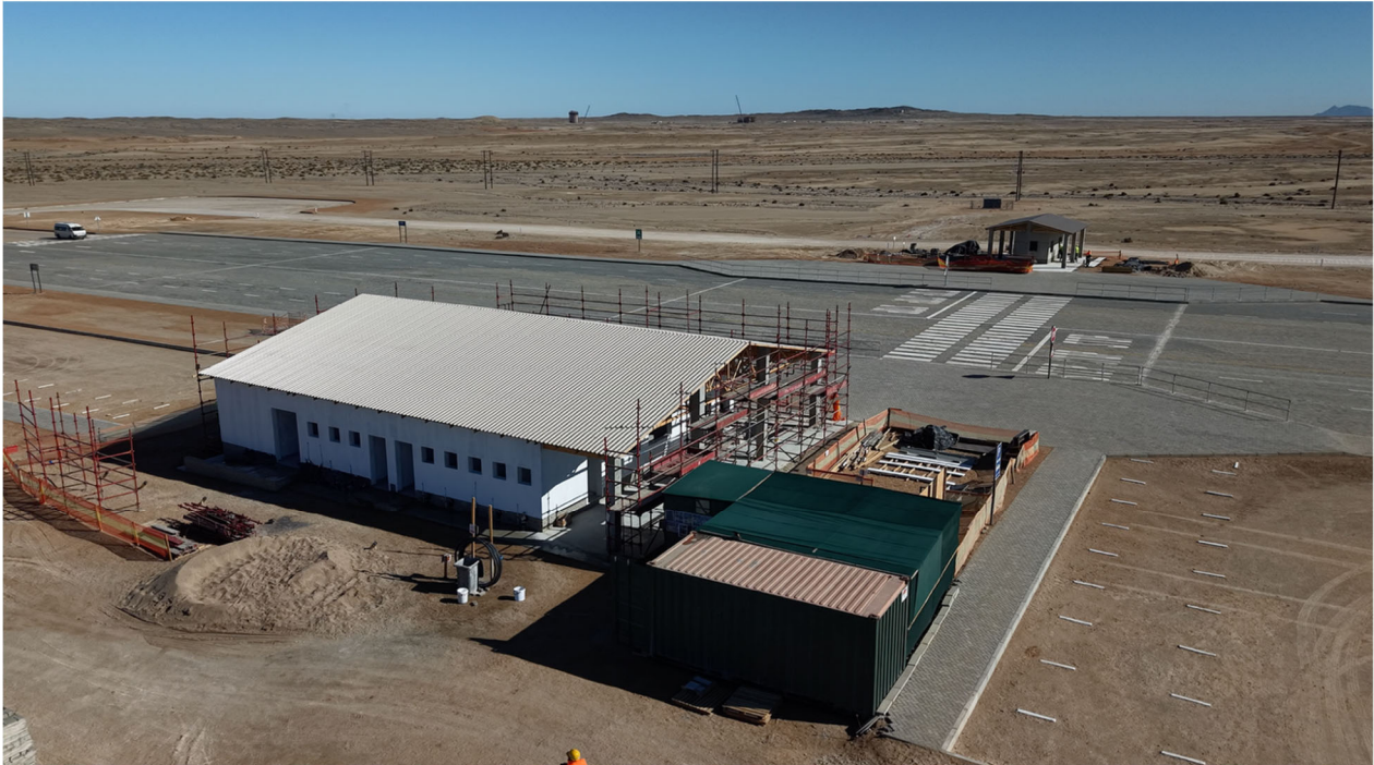
Figure 5: The gate house has continued to progress.
