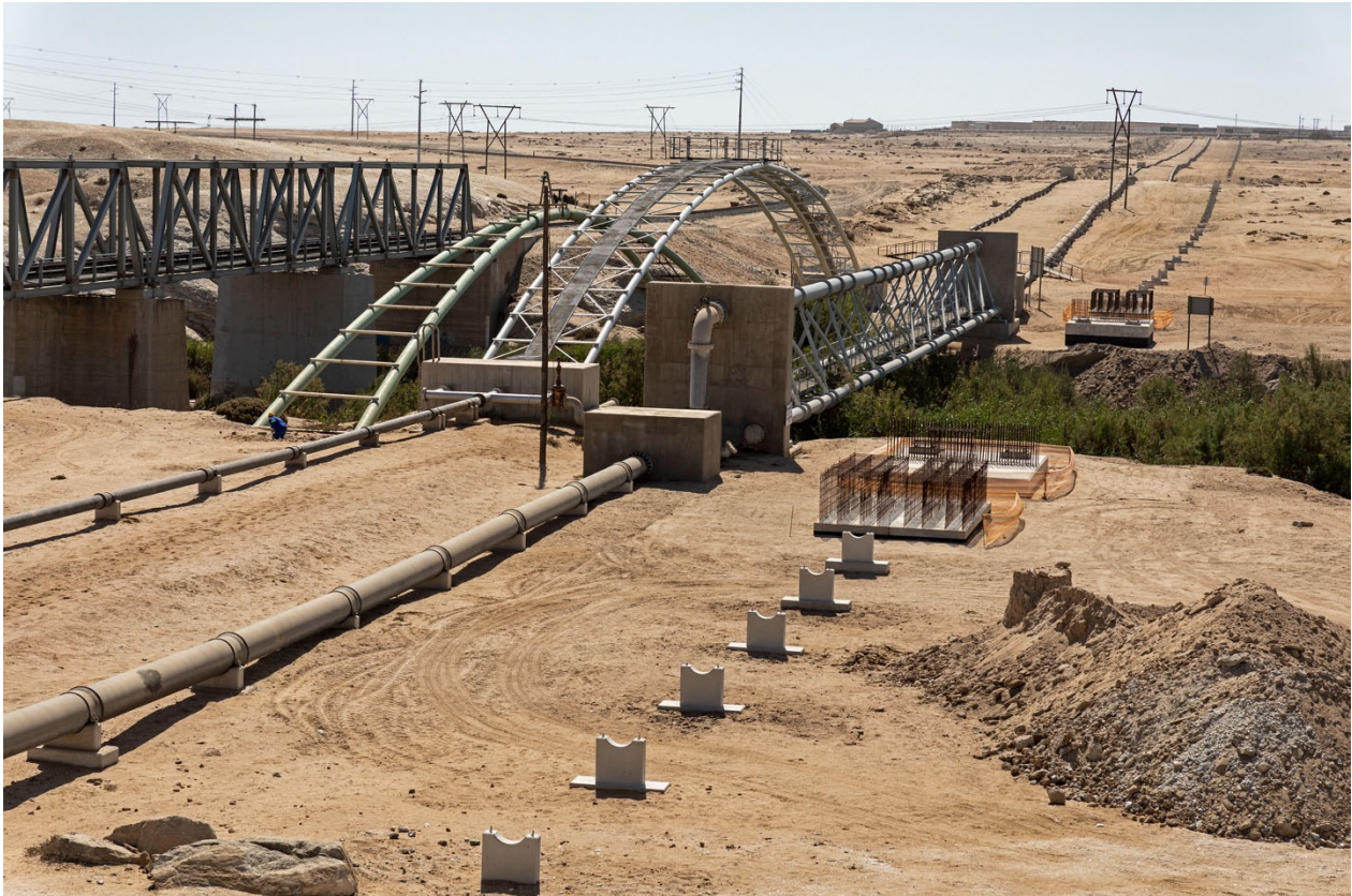
Figure 6: View of the Etango water pipeline pipe pedestals and foundations for the pipe bridge installation at the Swakop River crossing.
