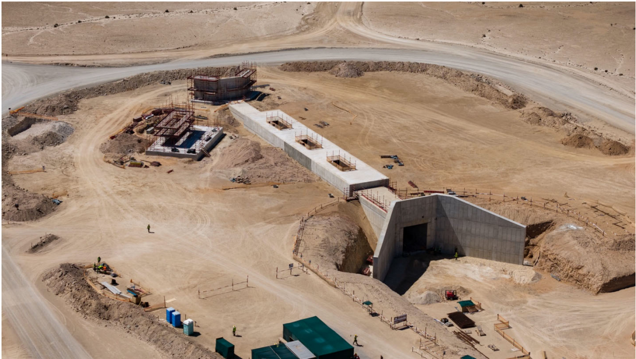
Figure 3: Aerial view of the stockpile tunnel where the roof and wing walls are now complete.
