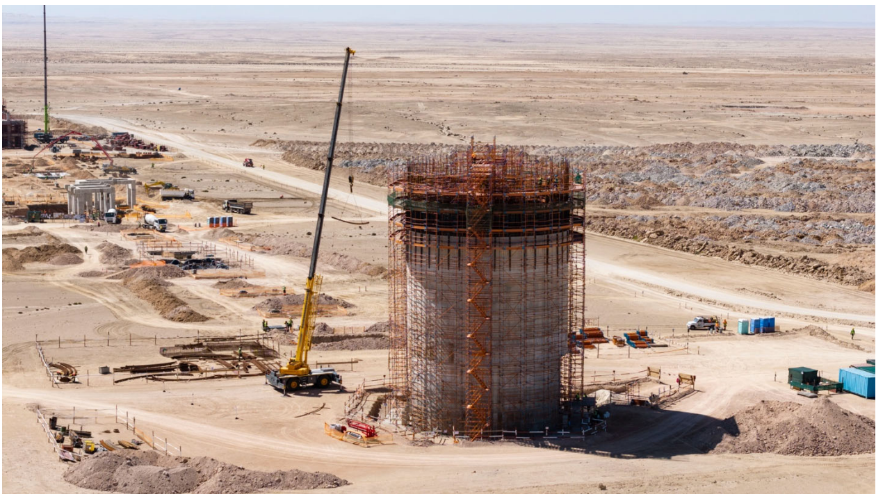
Figure 4: Aerial view of fine ore silo.
