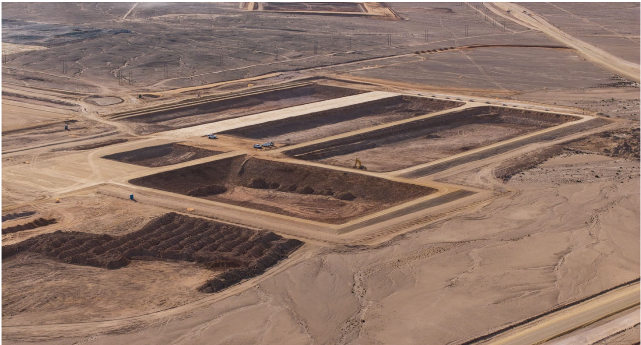
Figure 1: The wet plant terraces and solution ponds have progressed significantly.
