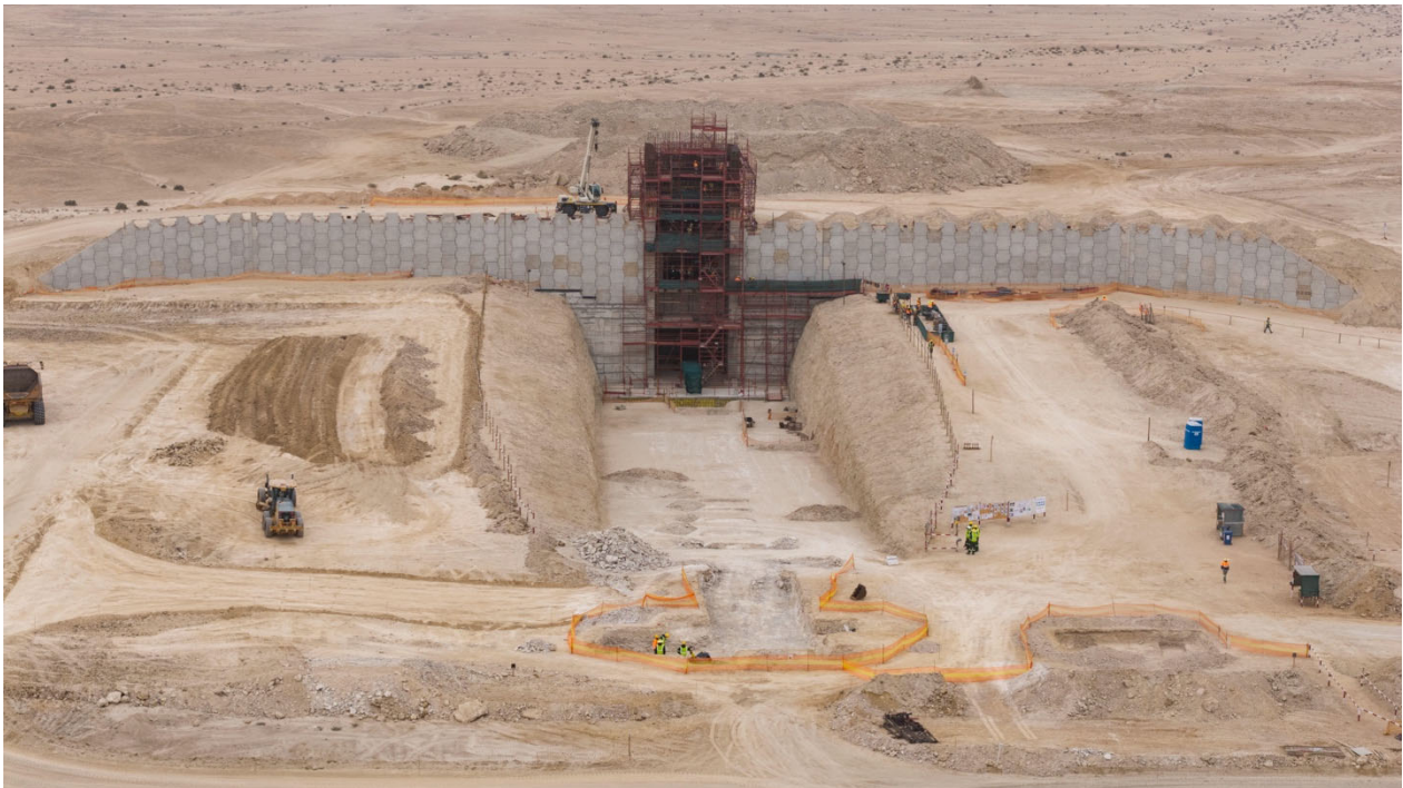
Figure 2: The primary crusher concrete structure is being advanced concurrently with the pre-cast retaining wall installation
