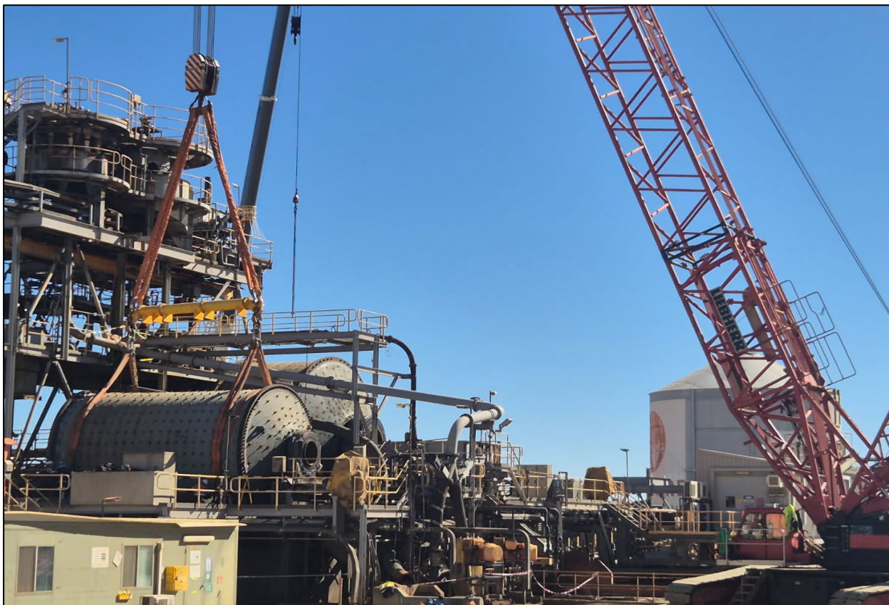
Photo 7: Ball Mill Removal at DeGrussa
