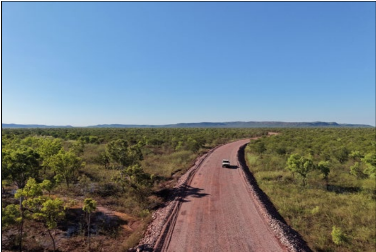
Photo 1: Main Access Road Constructed
