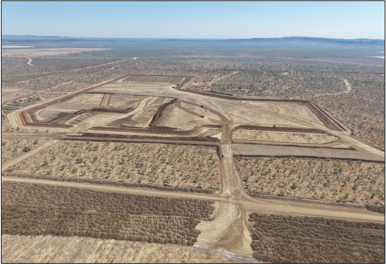
Photo 5: Evaporation Pond Construction Underway
