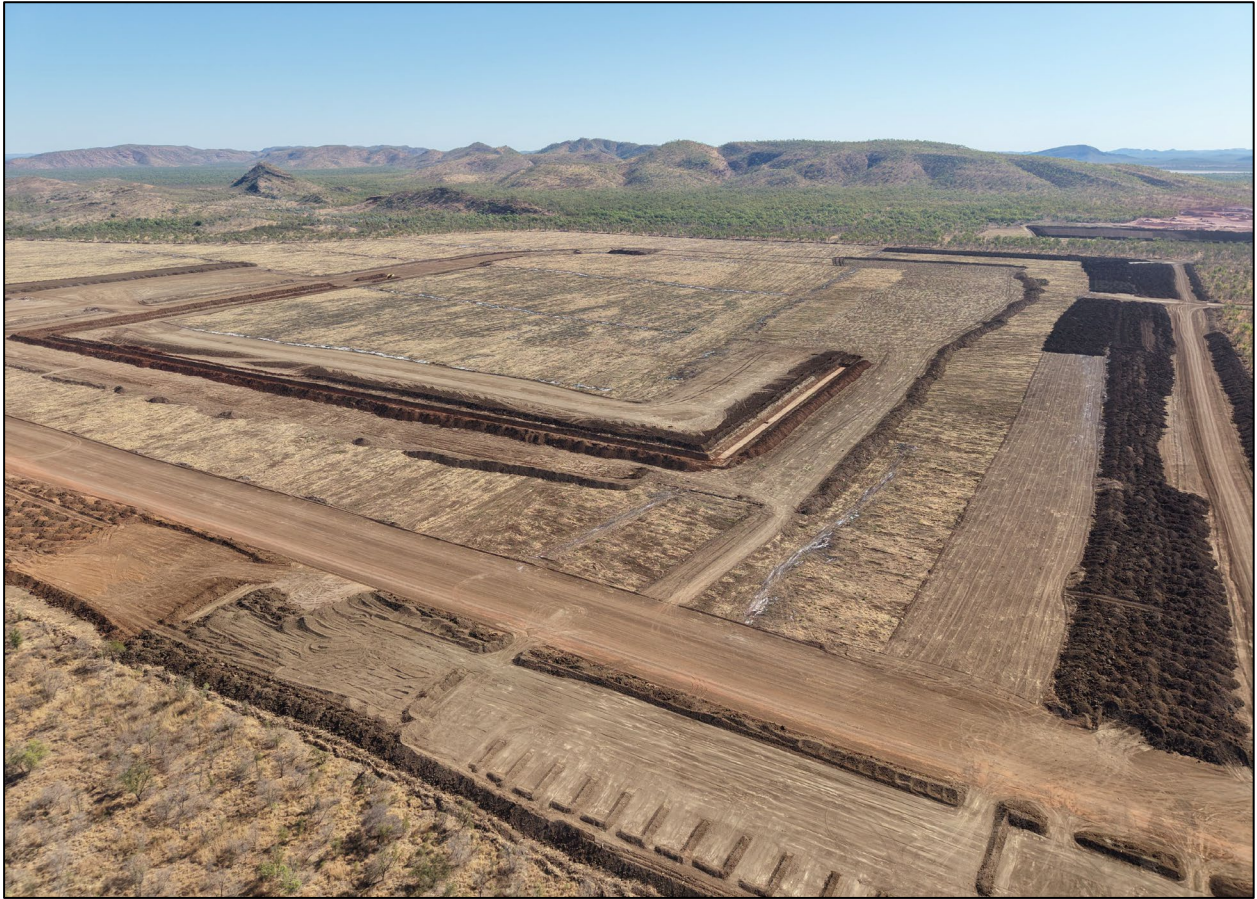
Photo 3: Tailings Storage Facility Construction Underway
