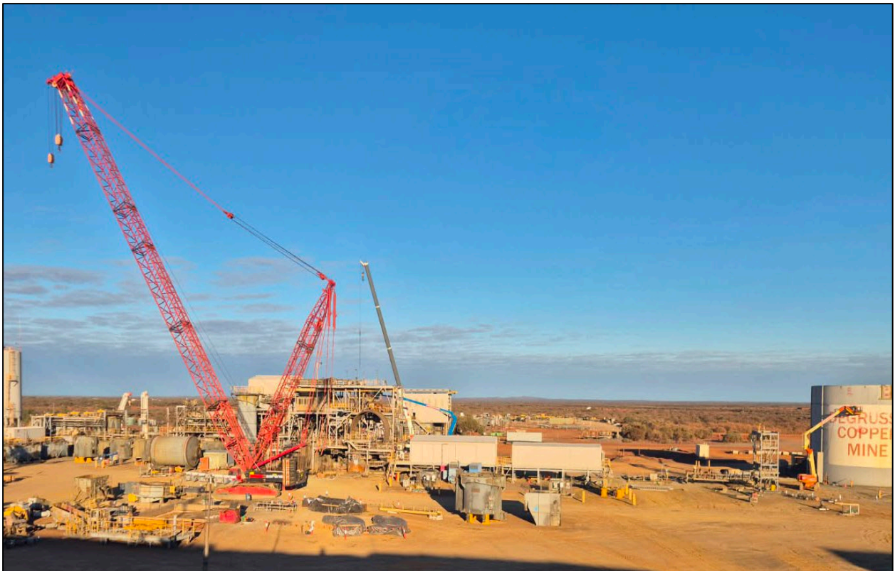
Photo 6: Grinding and Flotation Area Deconstruction at DeGrussa
