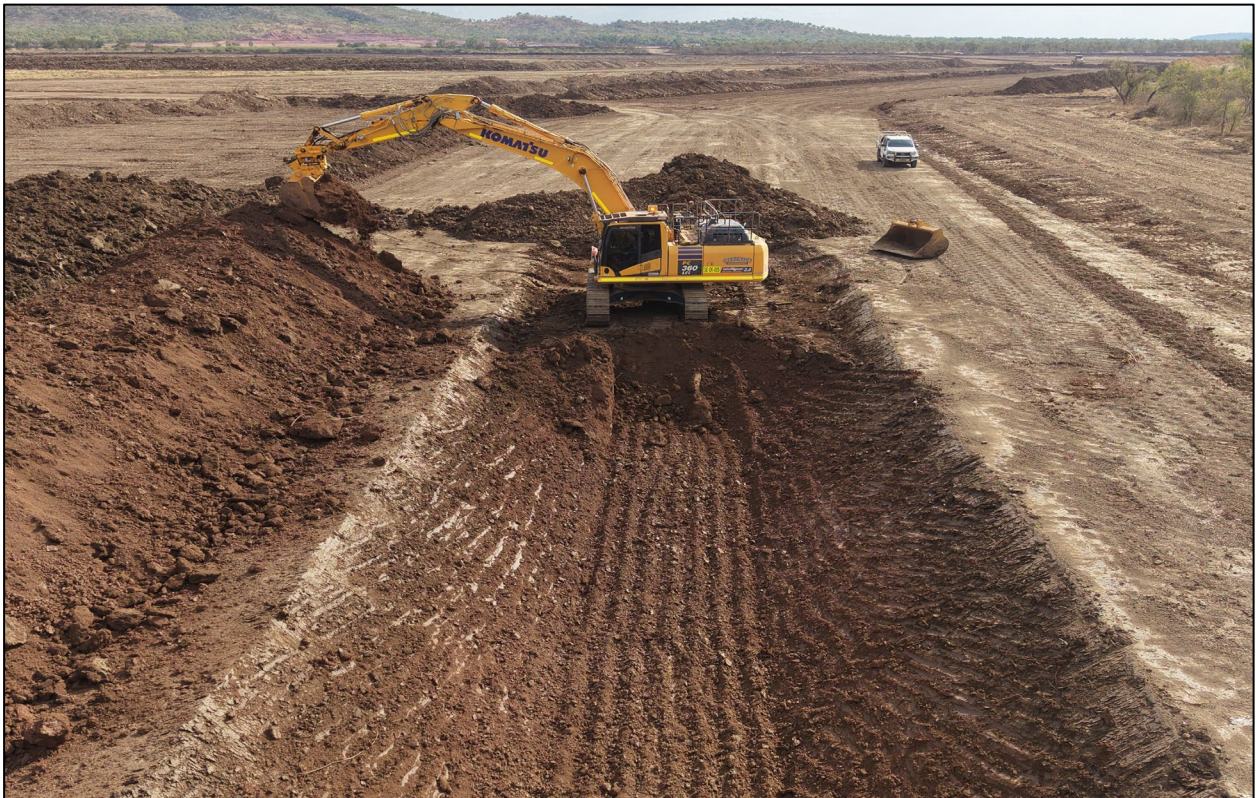
Photo 4: Keyway Excavation in Tailings Storage Facility
