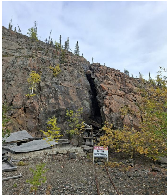
Figure 7. Adit/mine opening at the foot of the vein, with remnant rail, looking ENE.
