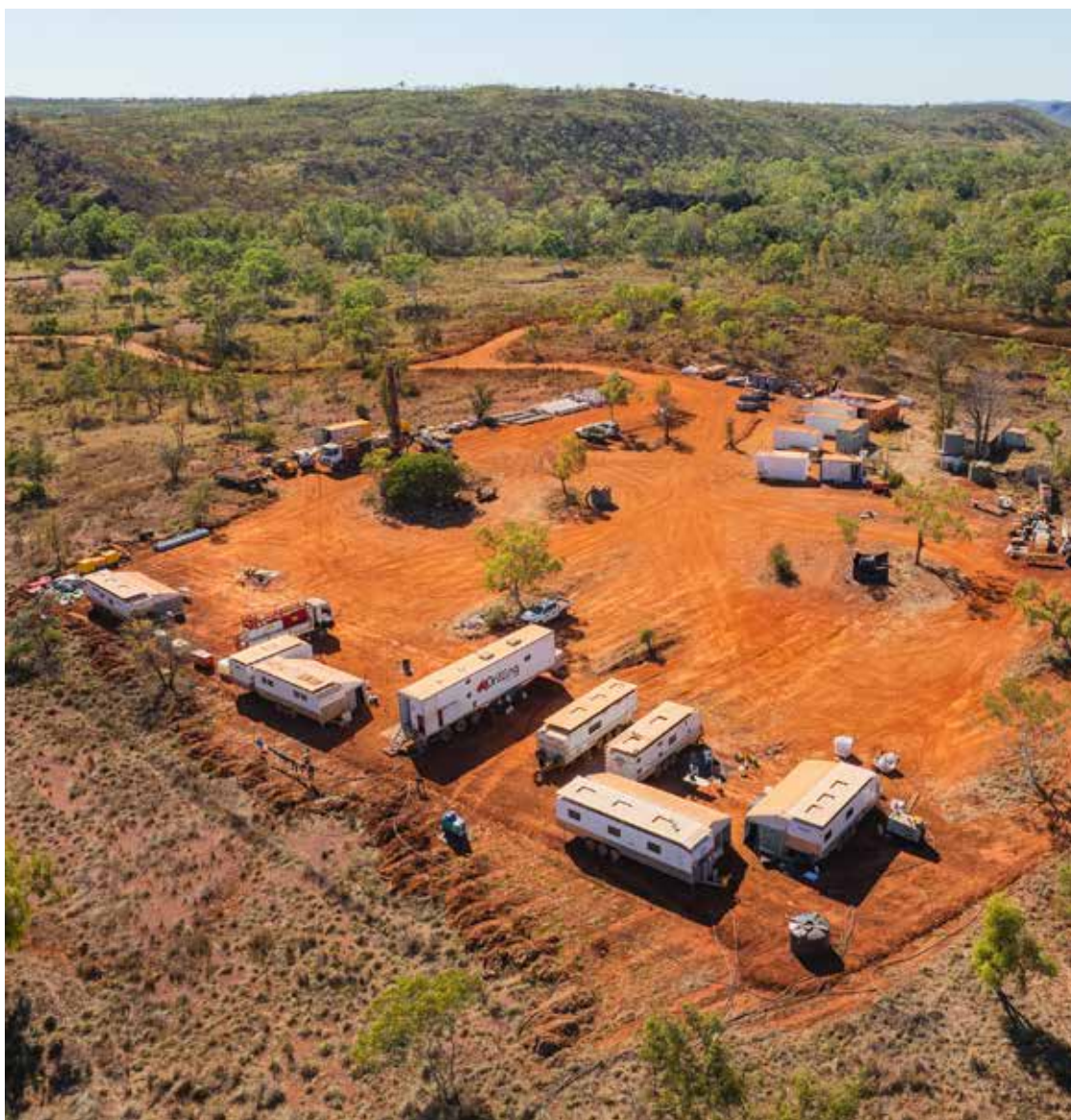
Speewah Fluorite Project site facilities
