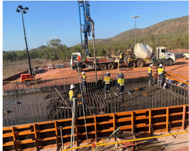
Figure 3: Process Plant Civil Works at Sorby Hills
