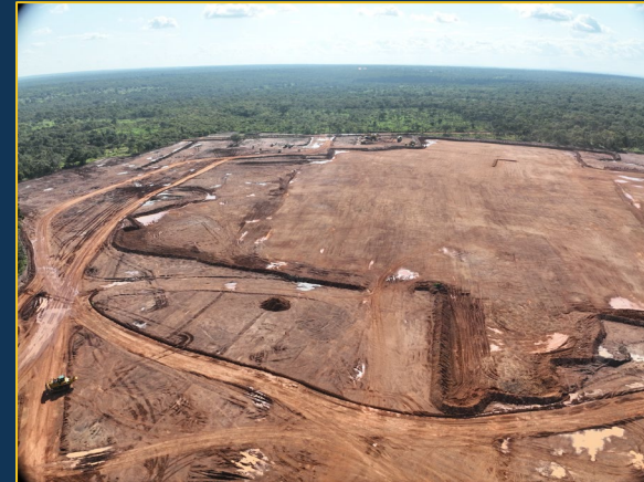
Process Plant Earthworks
