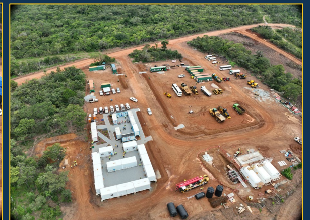
Contractor Laydown & construction Offices
