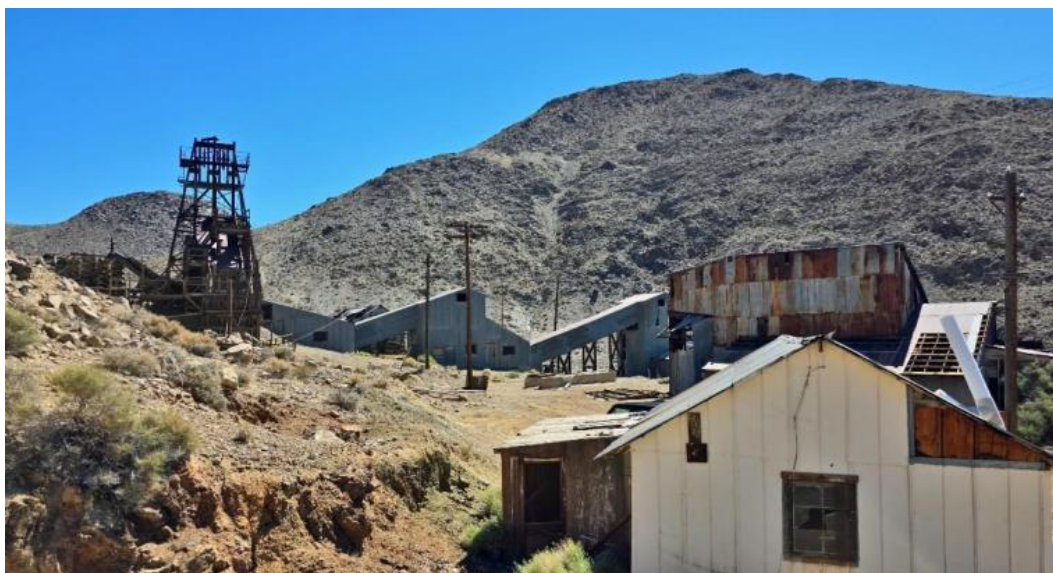
Figure 1. Historical headframe, mill buildings and surface infrastructure at Nevada Scheelite, looking northeast.
