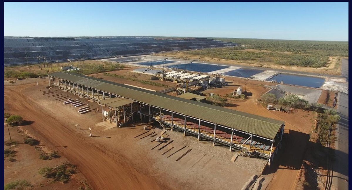
Mt. Kelly Heap leach and processing facility from the air
