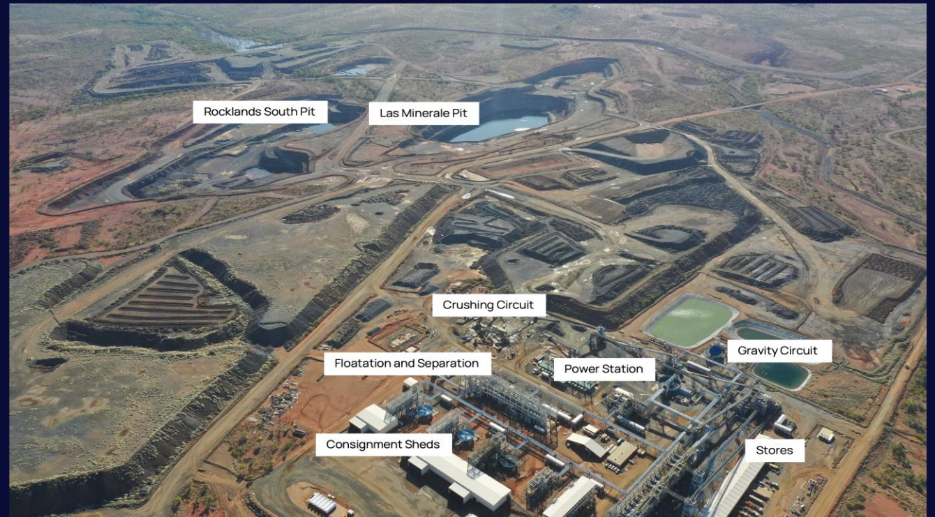
Rocklands processing facility from the air
