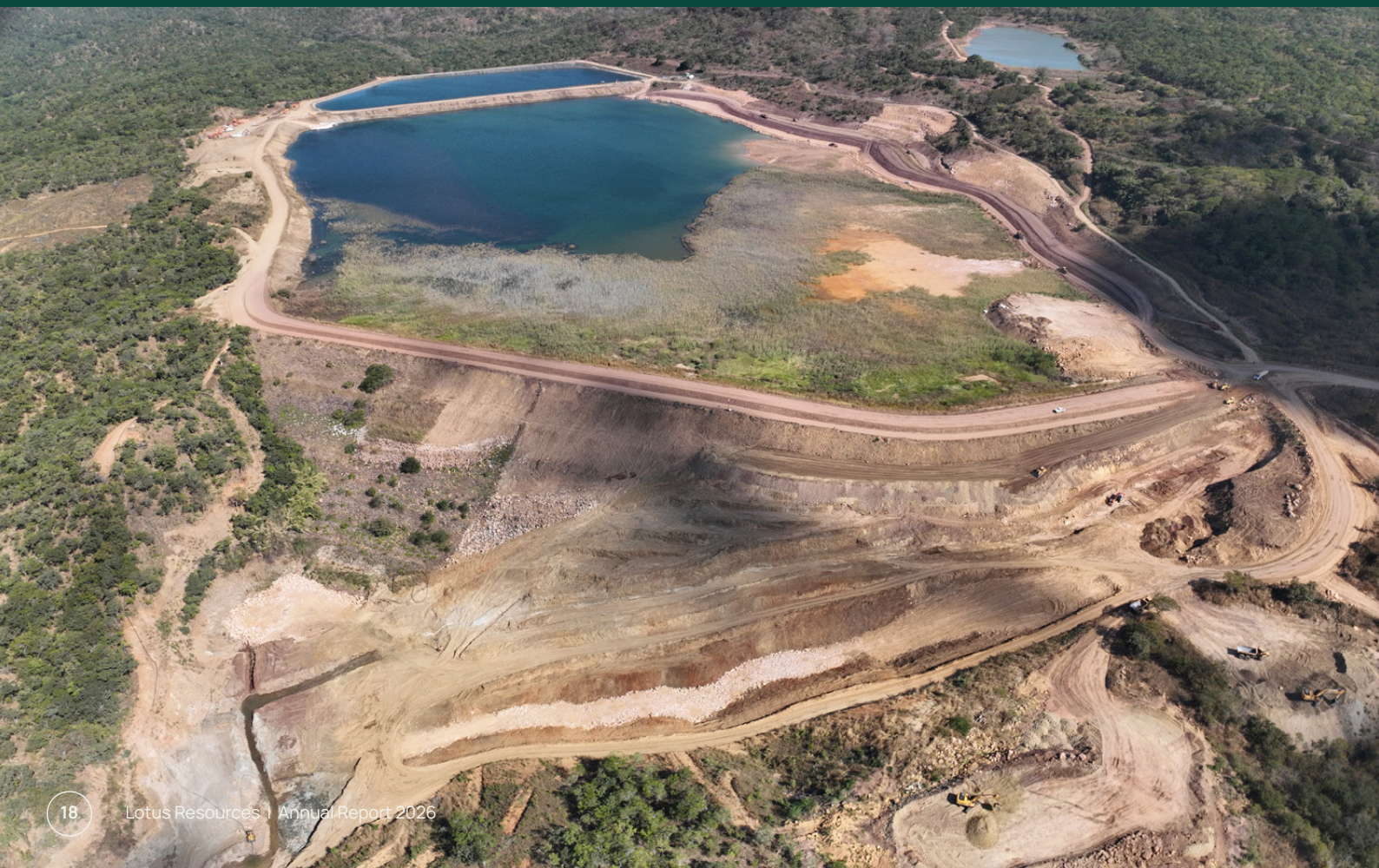
Figure 5: TSF expansion works, June 2026
