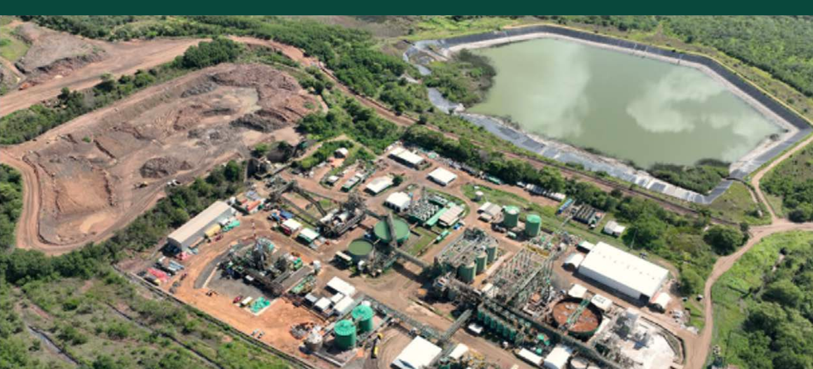
Figure 2: Kayelekera ROM pad, process plant and process water pond
