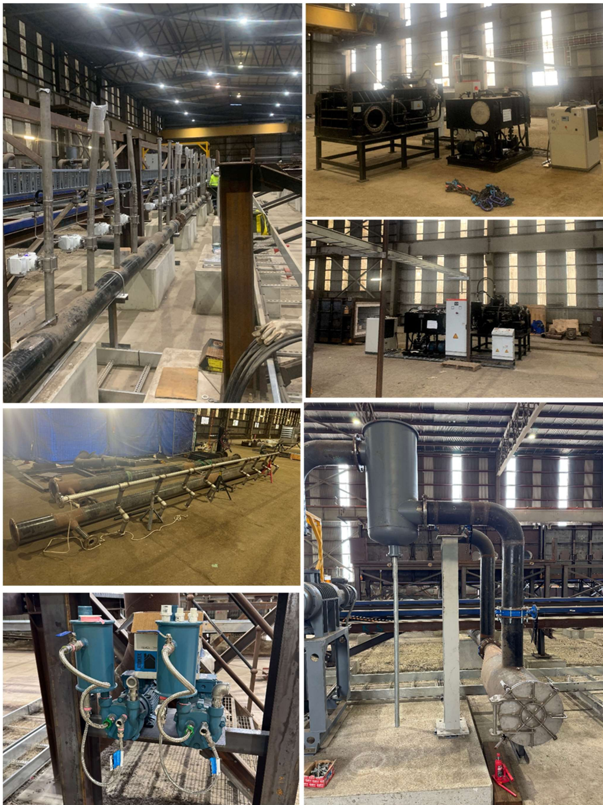
Figure: Vacuum piping manifold fabrication and piping installation, along with Baler installation progress.
