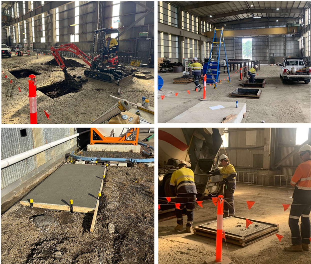
Figure: AMEC Industries mobilised to complete remaining civil scope.
