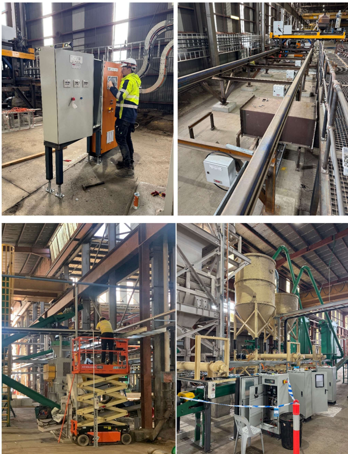
Figure: Reduction Furnace local junction boxes & main panel installation progress and Briquetting terminations complete and initial pre-testing of electrical equipment.
