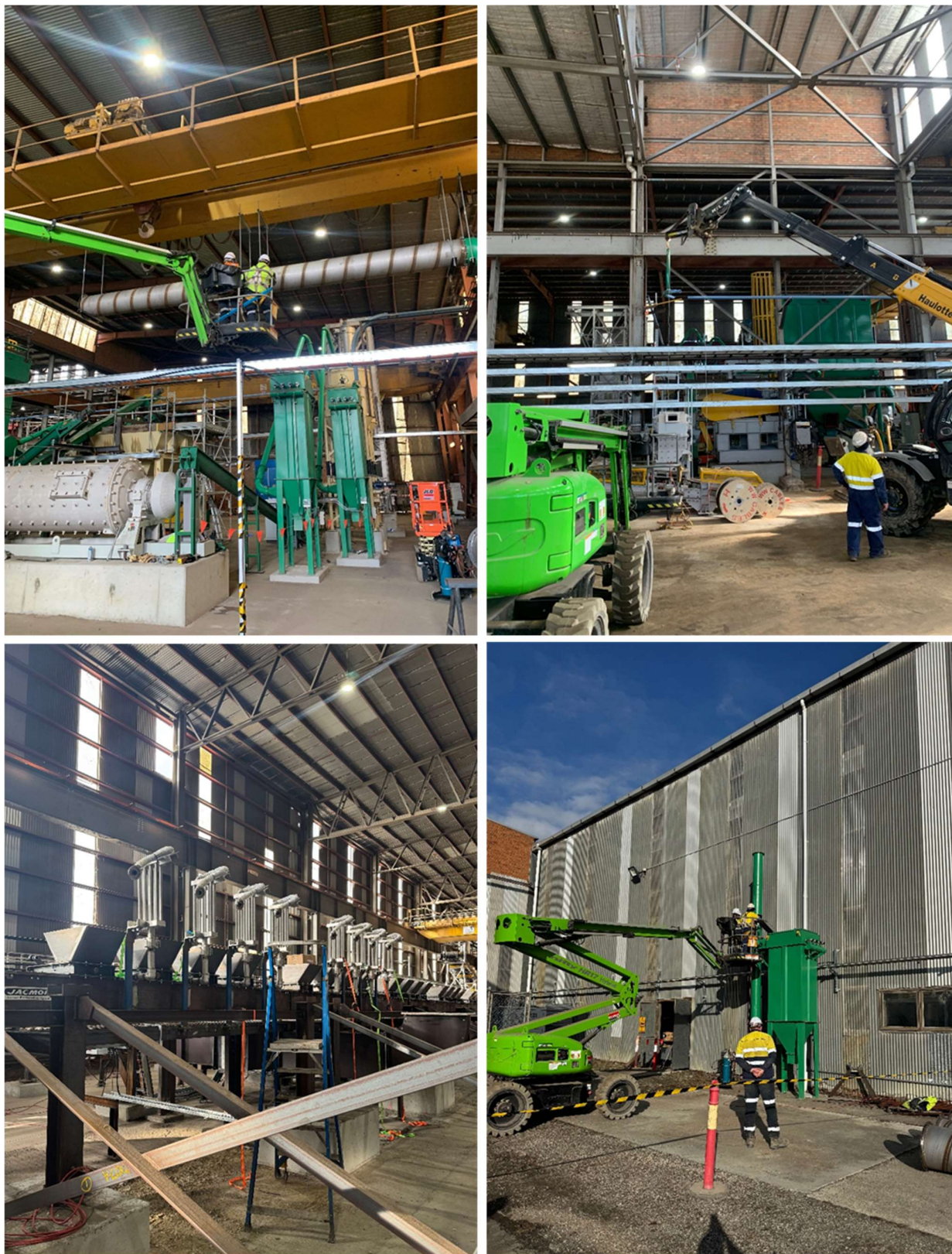
Figure: Ducting, reagent piping & Reduction Furnace vacuum piping installation progress.
