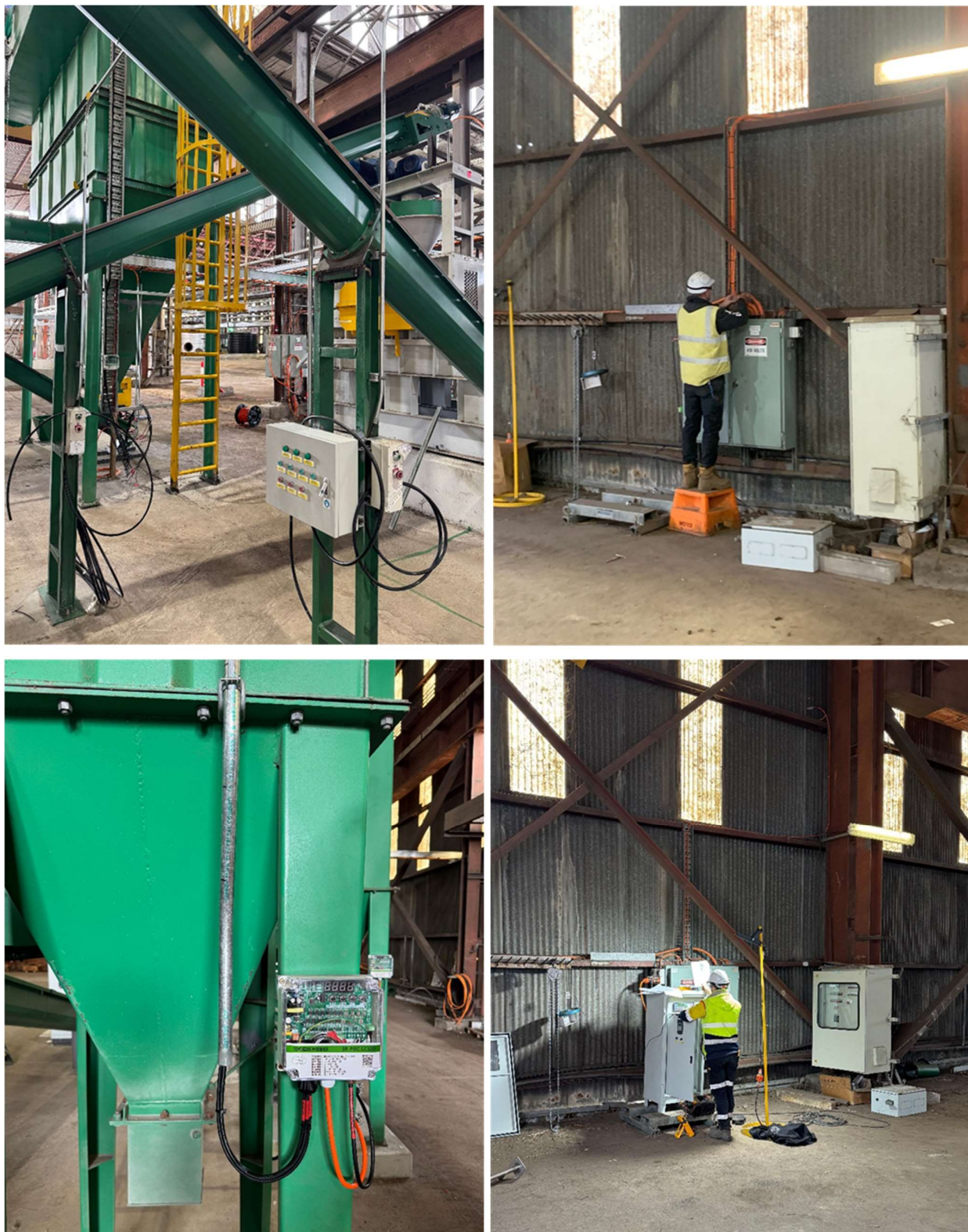
Figure: Briquetting electrical and instrumentation cable terminations progress.
