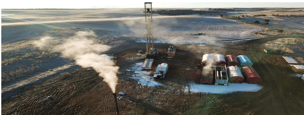
Figure 5: Jesse-1A flow test venting reservoir gases and helium through the flare stack.
