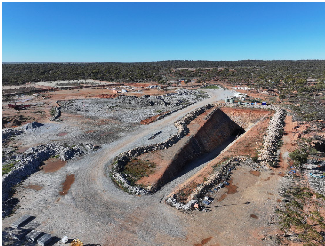
Figure 2: Radio boxcut and portal overlooking the proposed ROM and processing area
