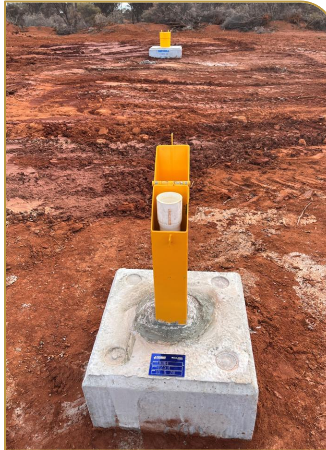
Production bore background and monitoring bore foreground
