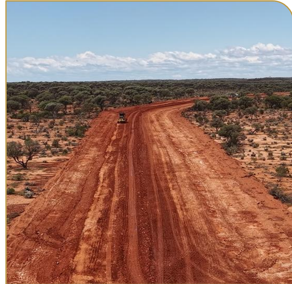
Mt Ida public road diversion commenced
