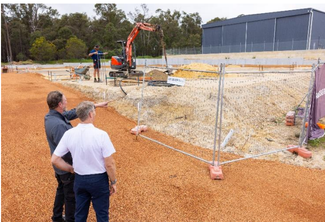
Fig 1: Construction in progress at Collie.
