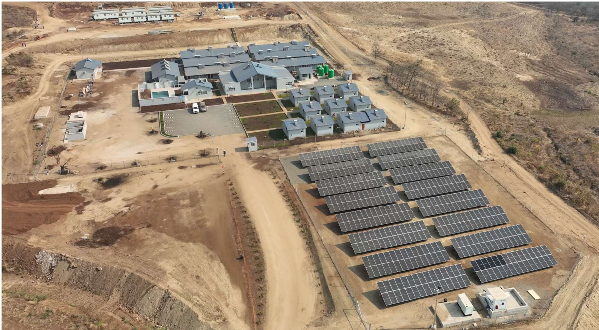
Picture 7. The fully operational Tipume Accommodation Camp and solar installation, supporting the site workforce
