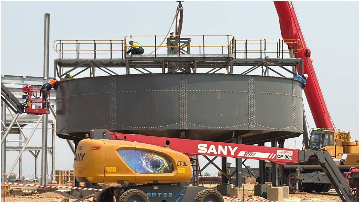
Picture 5. Thickener infrastructure substantially complete at the process plant area
