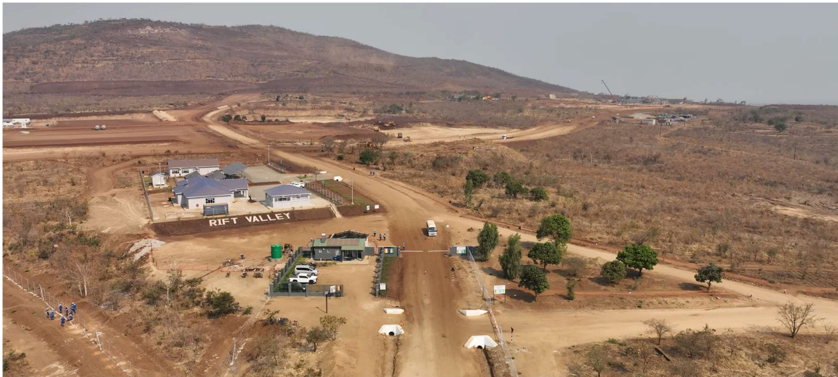
Picture 1. Kangankunde site access gate and administration precinct
