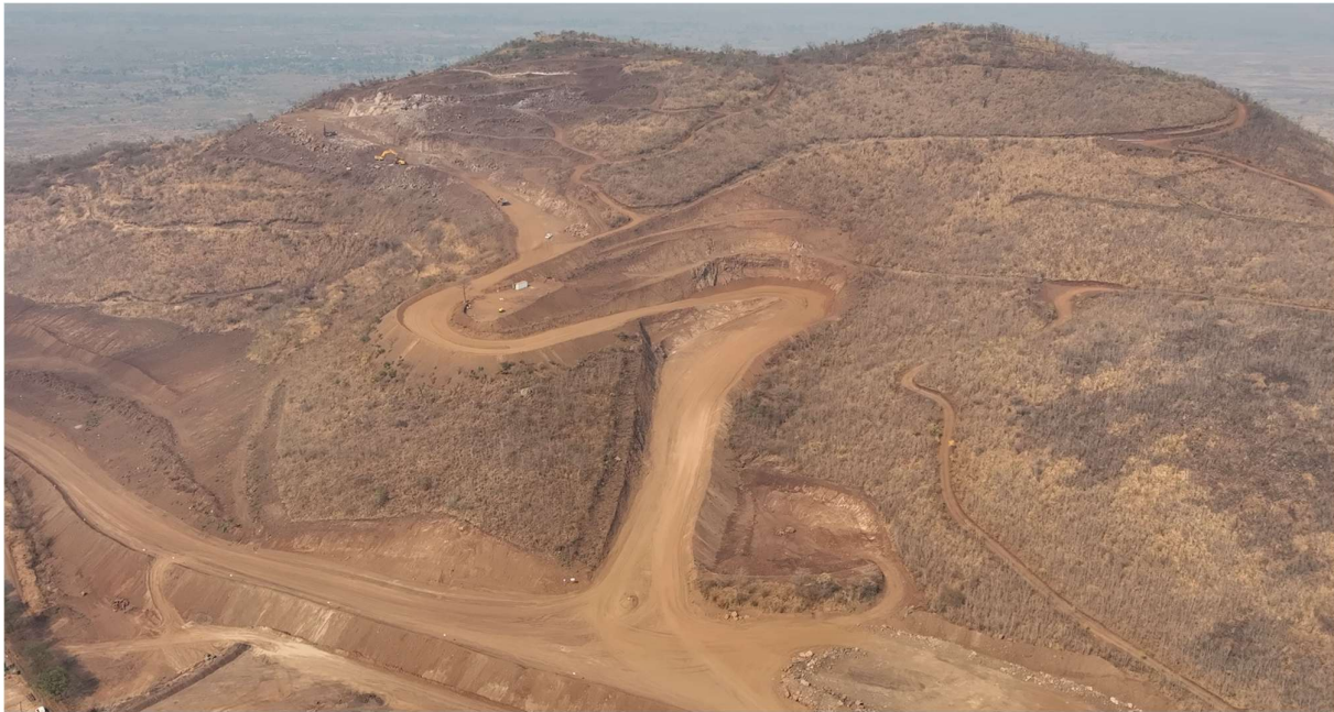
Picture 4. The opened Stage 1 pit and completed haul road at Kangankunde
