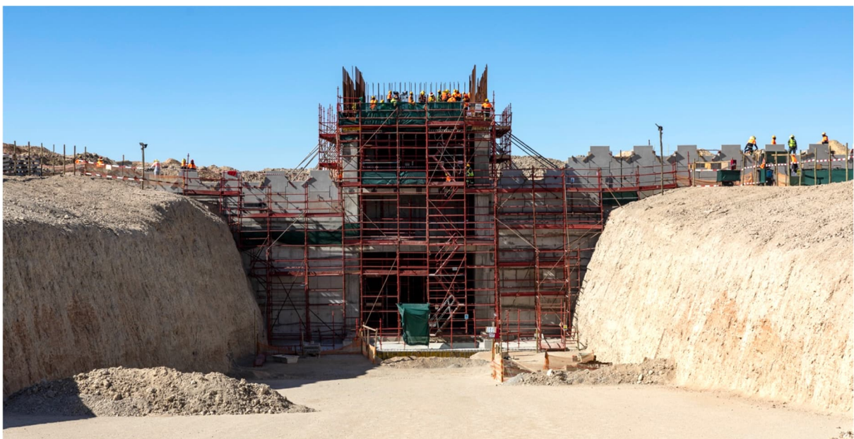
Figure 3: Structural concrete for the primary crusher progressed above ground level during the year.
