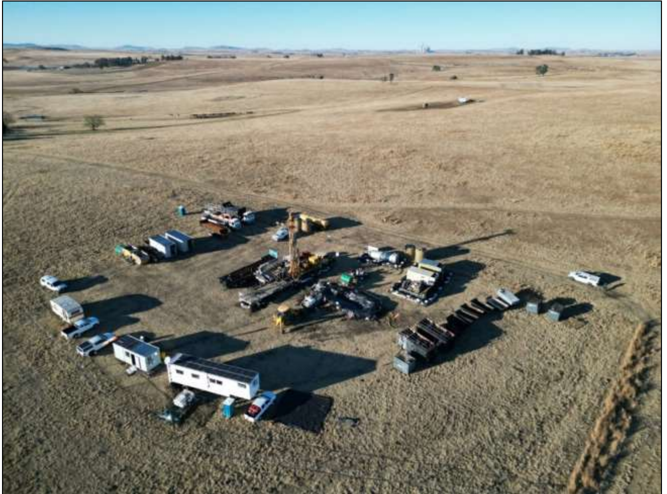
Figure 2 – Drilling rig on site for commencement of drilling at well 271-KA03PT06, Brakfontein.
