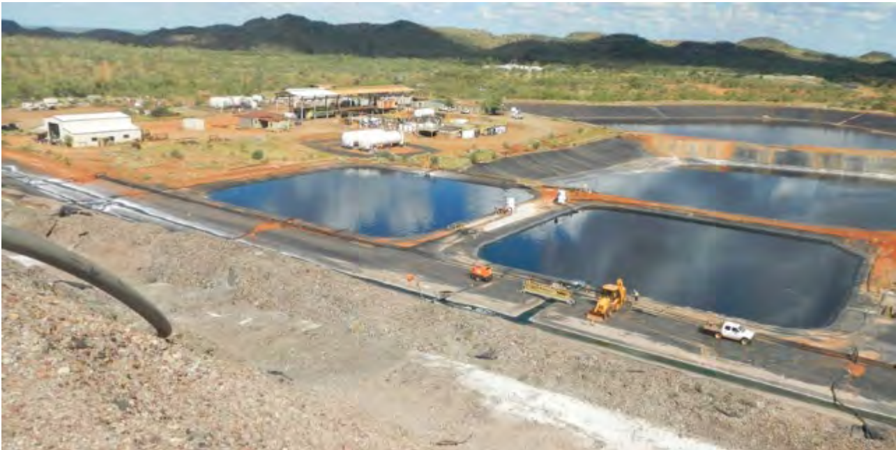
Figure 7-2. Mt Cuthbert SX-EW processing plant and adjacent ponds as at March 2022.
