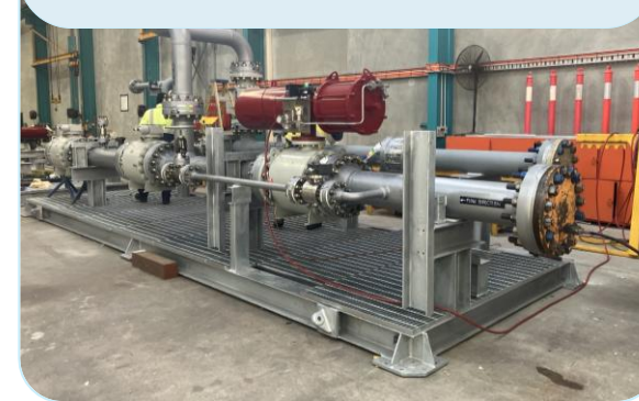
WPF Skid Fabrication - Waitsia 2B
