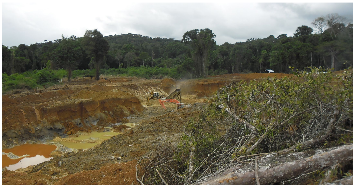
Figure 9 – Excavator-assisted workings on the Gonini Project with small-scale pump-and-sludge operation on the pit floor [circa 2020].
