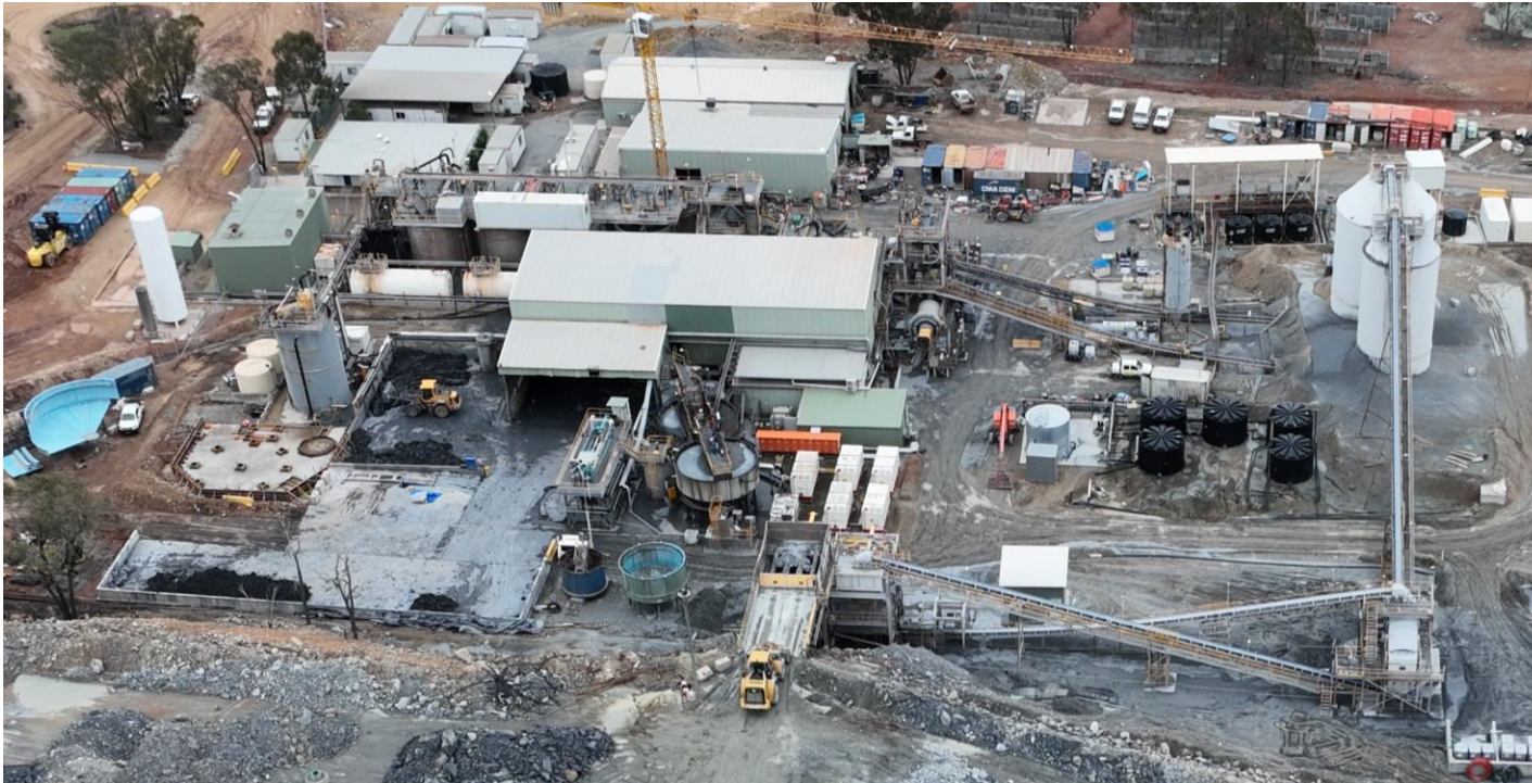
Processing plant and mine infrastructure
