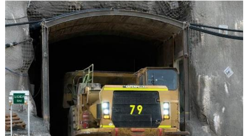
Eastern decline portal
