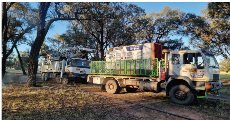
Figure 1: Drill rig mobilising at the Gilmore Project (21 September 2026).
