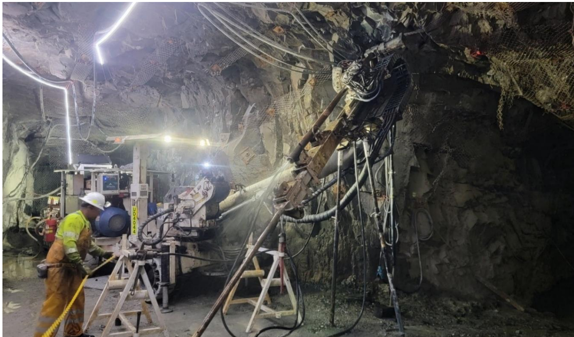
Figure 1: Drilling of DDH0294 commenced at cross-cut 11 (XC11), 17 September 2026 (PST).
