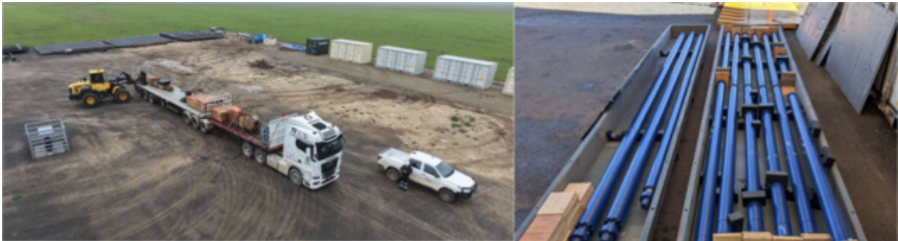
Figure 5 – Mobilisation and electric submersible pump equipment for the 2026 Ramsay flow-testing campaign.
