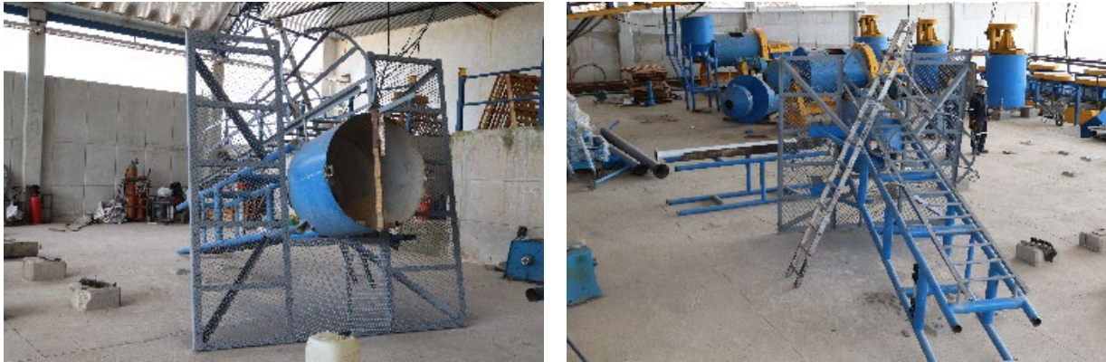
Figure 5: Cyclone tower construction
