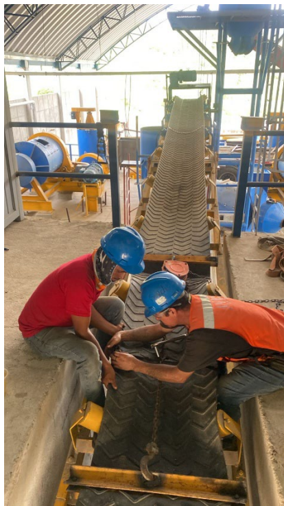
Figure 2: Conveyor to mill feed – belt refurbishment and installation of the mill feed conveyor
