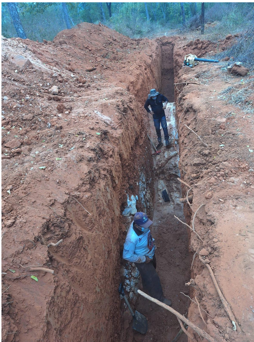
Figure 2: Channel sampling undertaken earlier in 2026 at Trench TR01, with exposed pegmatite shown towards the rear of the trench at the Mauricio Target, Igrejinha tenement, Brazil. 7
