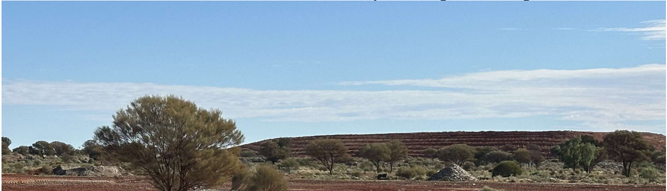
Photo 1: Minesite Rehabilitation of Neta Waste Dump showing contouring
