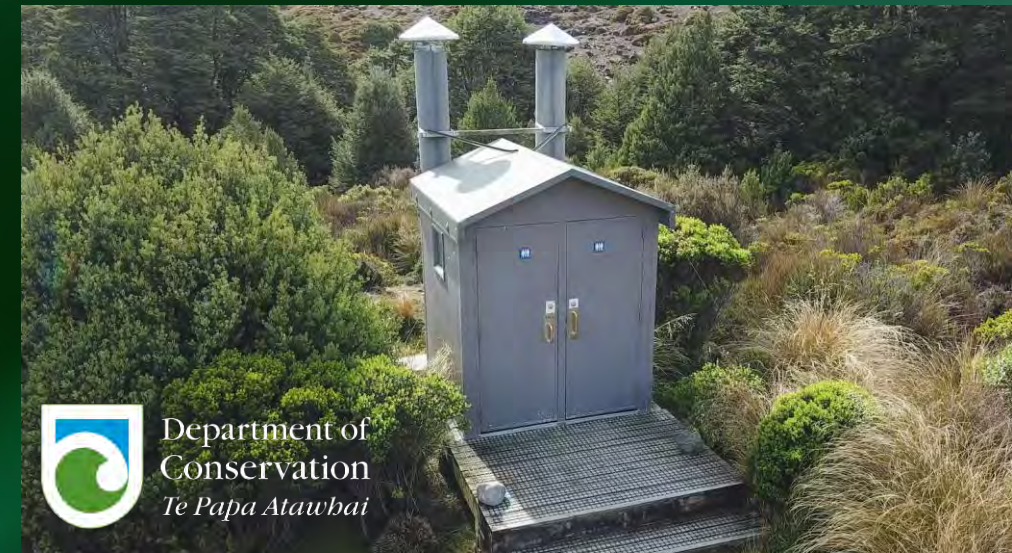
Example of an IoT-connected toilet
