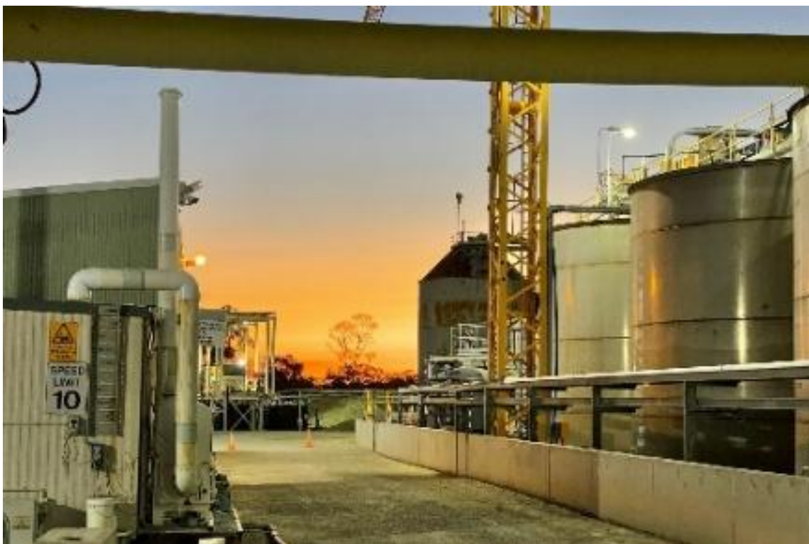
Figure 1: Mineral Hill processing plant.
