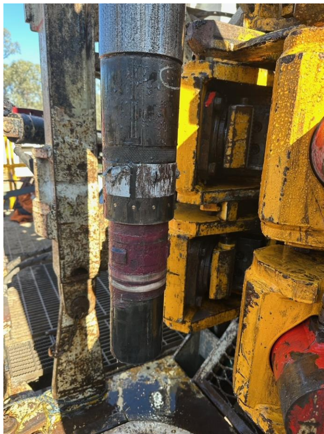
Image 1: Venus-2H: Liner release tool recovered to surface, leaving the liner in place within the well as preparations progress towards production testing.
