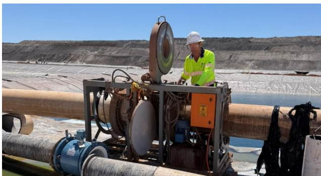
Welding main pipeworks
