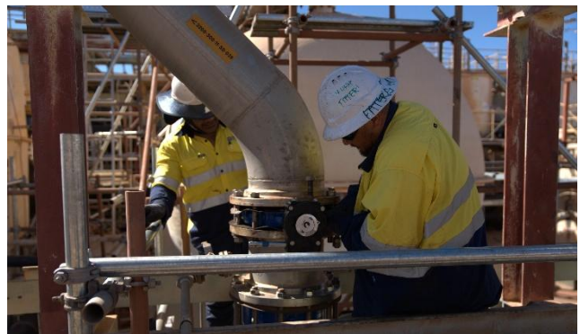
Detailed pipe installation
