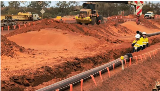
Process water lines being buried
