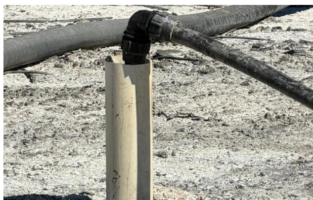
Low pressure injection during trial
