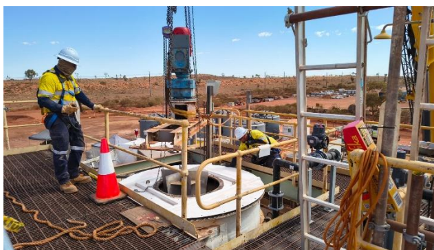
Mixer blade and rotor lifted and installed
