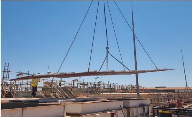
Settler tank lids lifted into place
