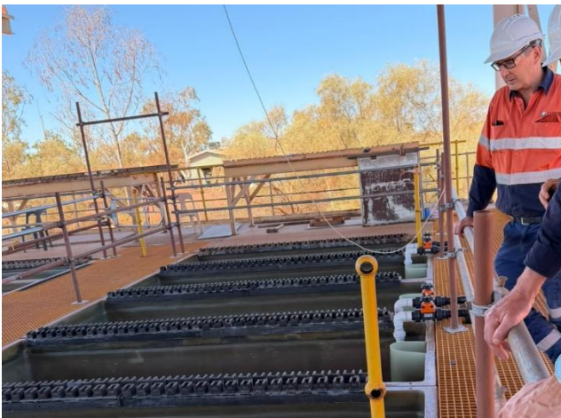
Cell top furniture being installed
