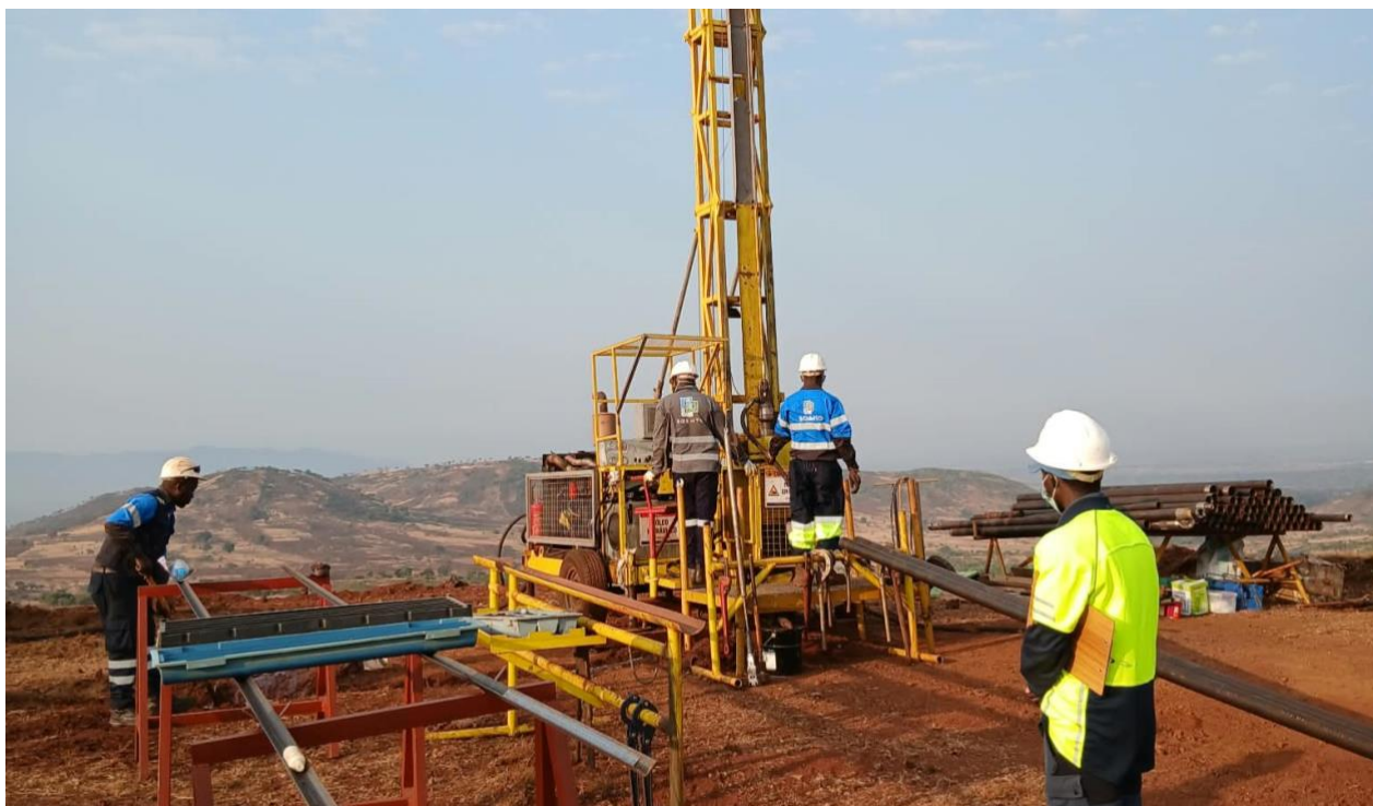
Figure 1 – Diamond drilling underway at primary Nb target
