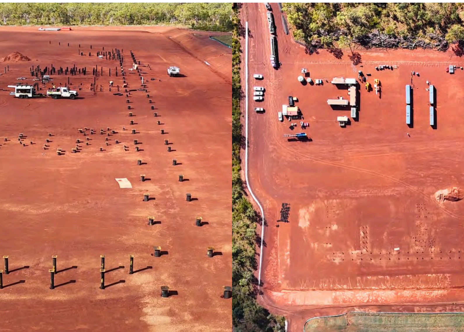
Installation of foundation piles at Carpentaria Gas Plant
