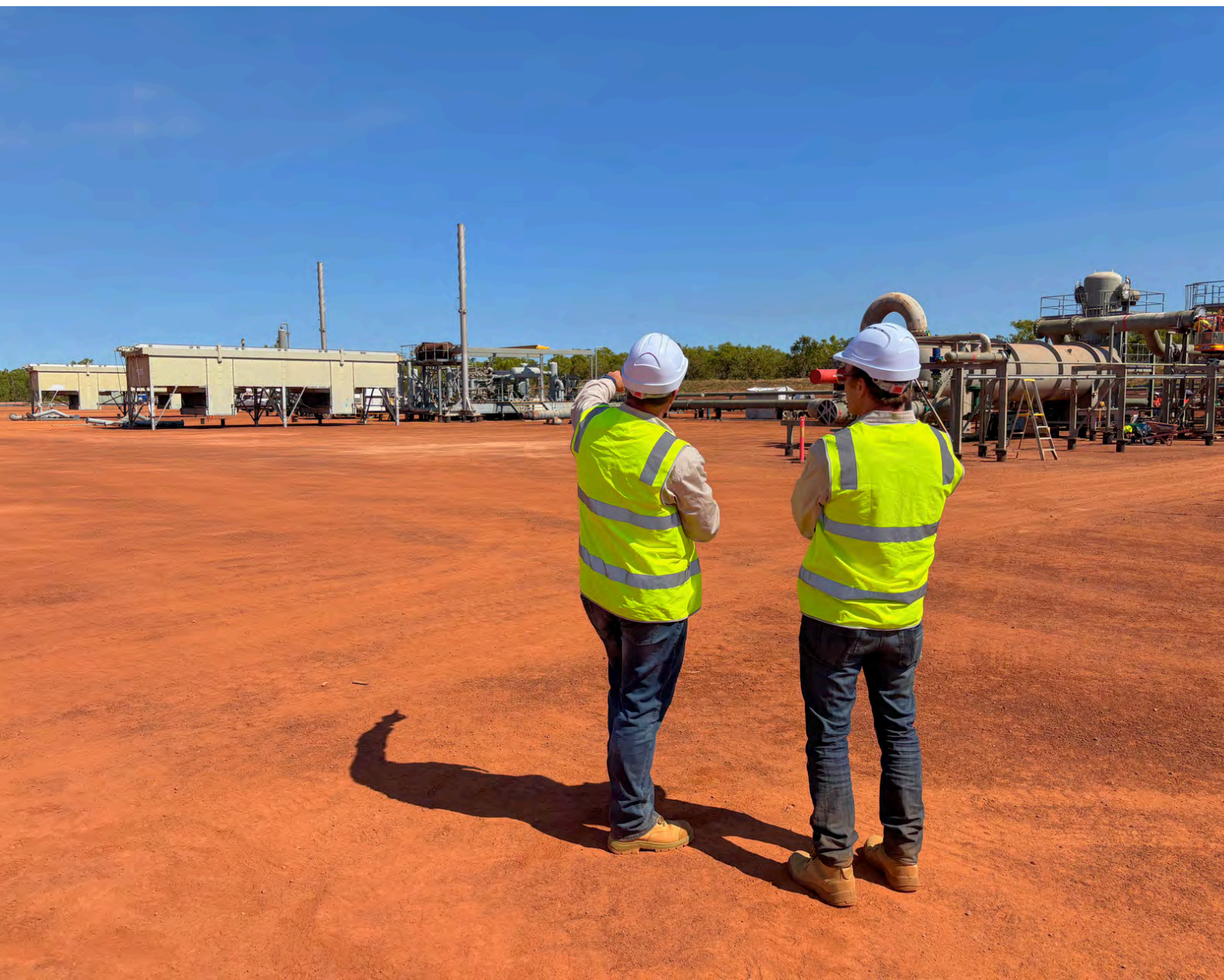
Carpentaria Gas Plant
