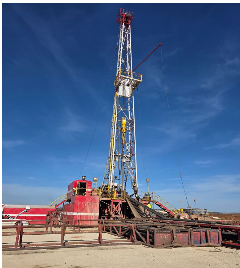
Photo 1: JVU-4 drilling operations at the Varn Oil Field
