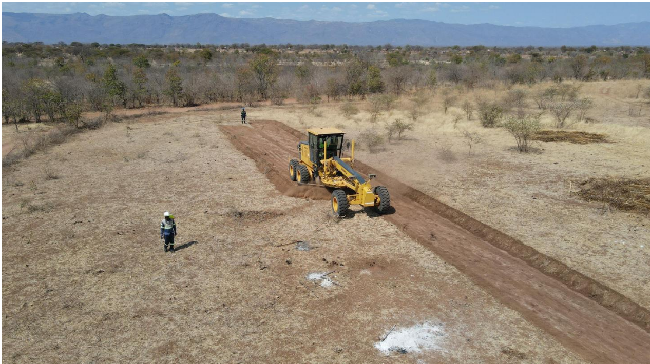
Figure 4 - Musuma-1 Wellpad ground breaking
