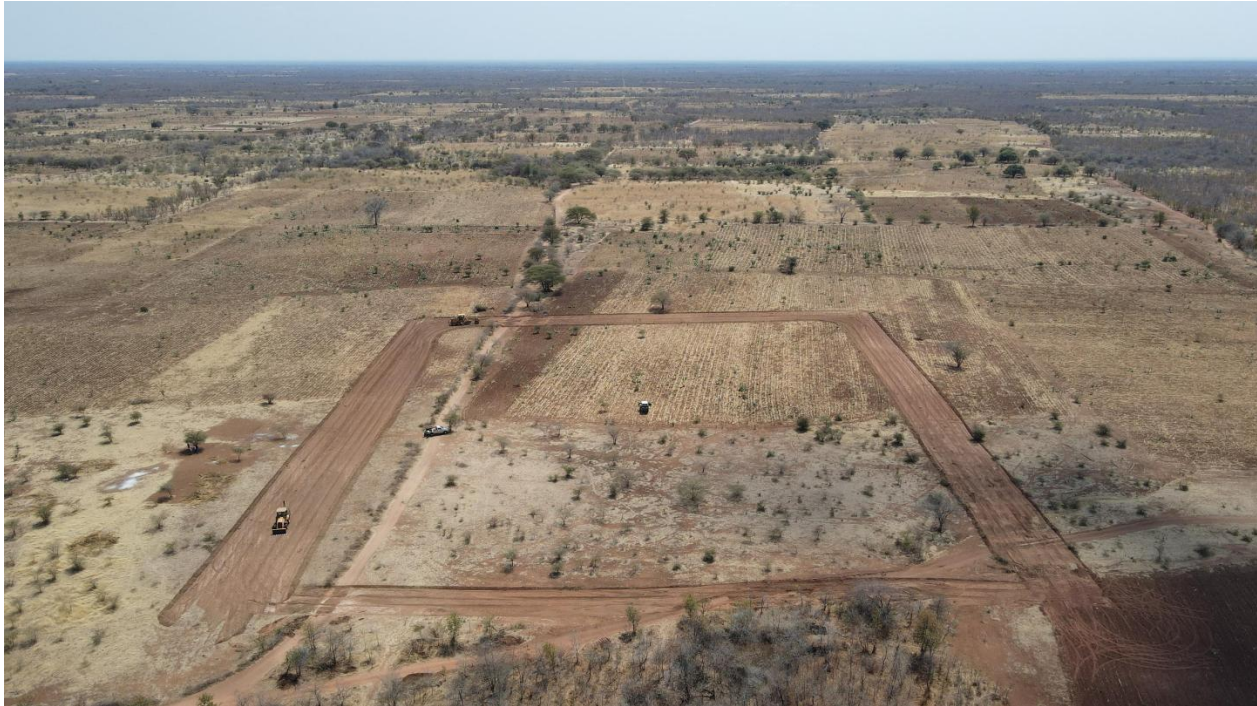
Figure 3 - Musuma-1 wellpad preparation
