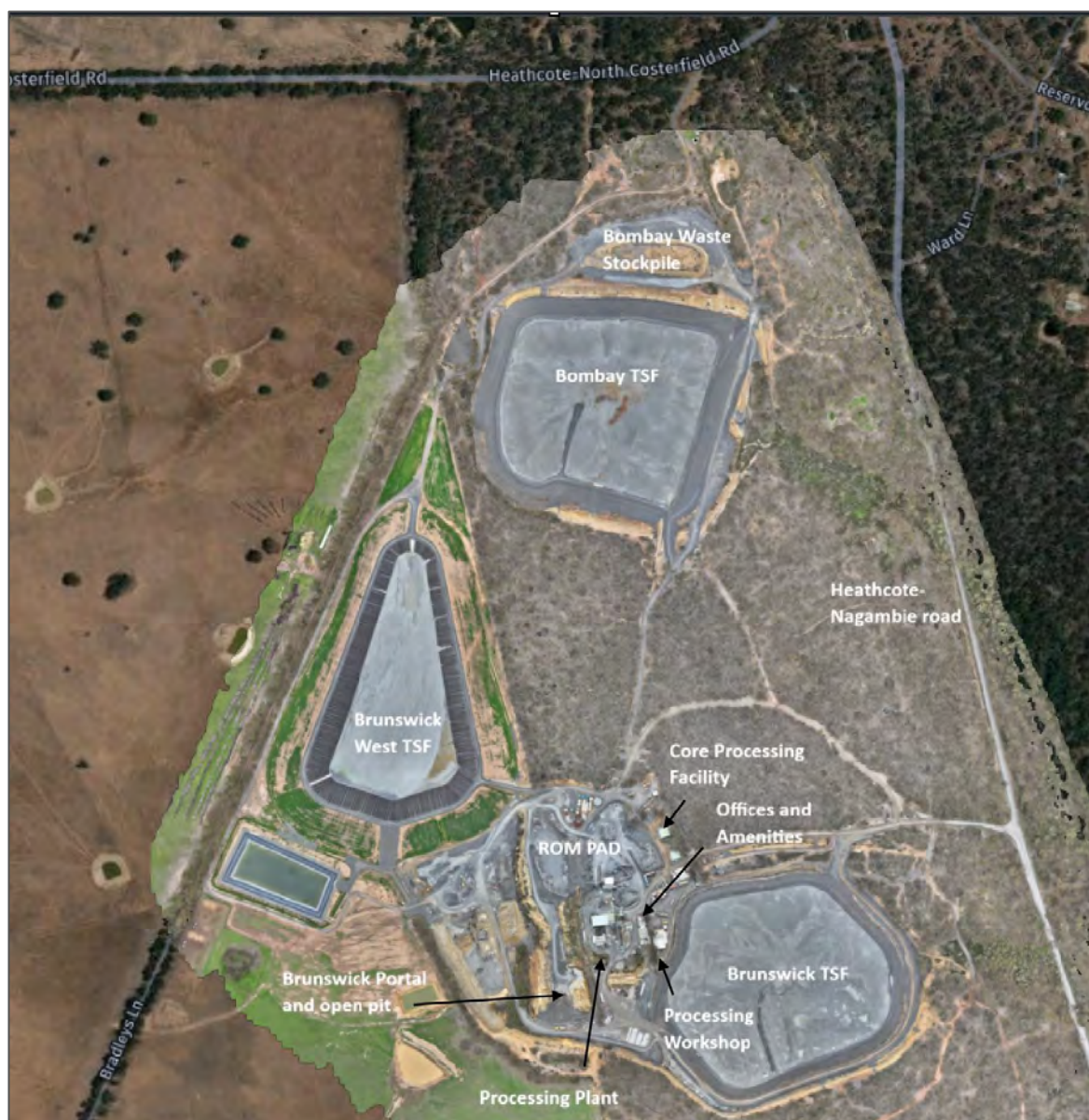
Figure 18.2: Brunswick Mine site – aerial view
