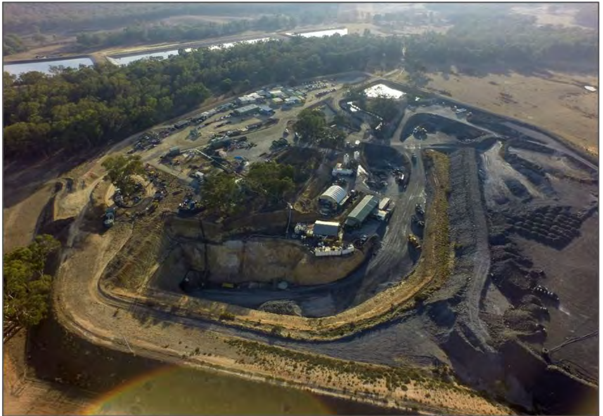
Figure 5.1: Augusta Mine site with box cut, Augusta Portal (foreground), workshop, offices and holding dams
