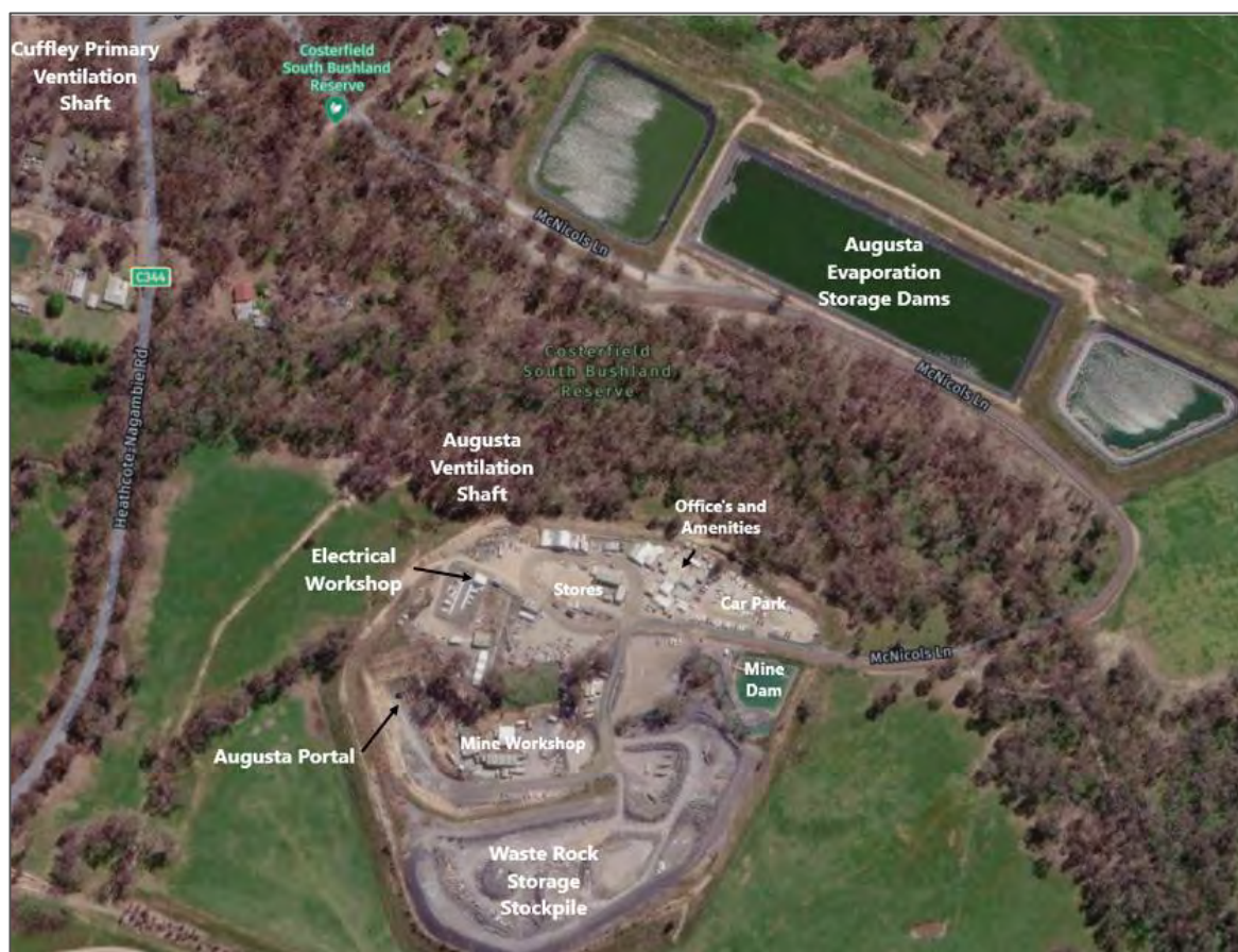
Figure 18.1: Augusta Mine site – aerial view
