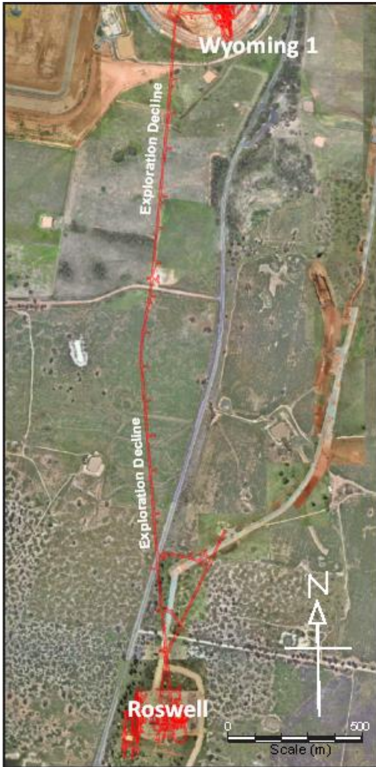
Figure 16-2: Exploration decline from Wyoming portal to Roswell orebody
