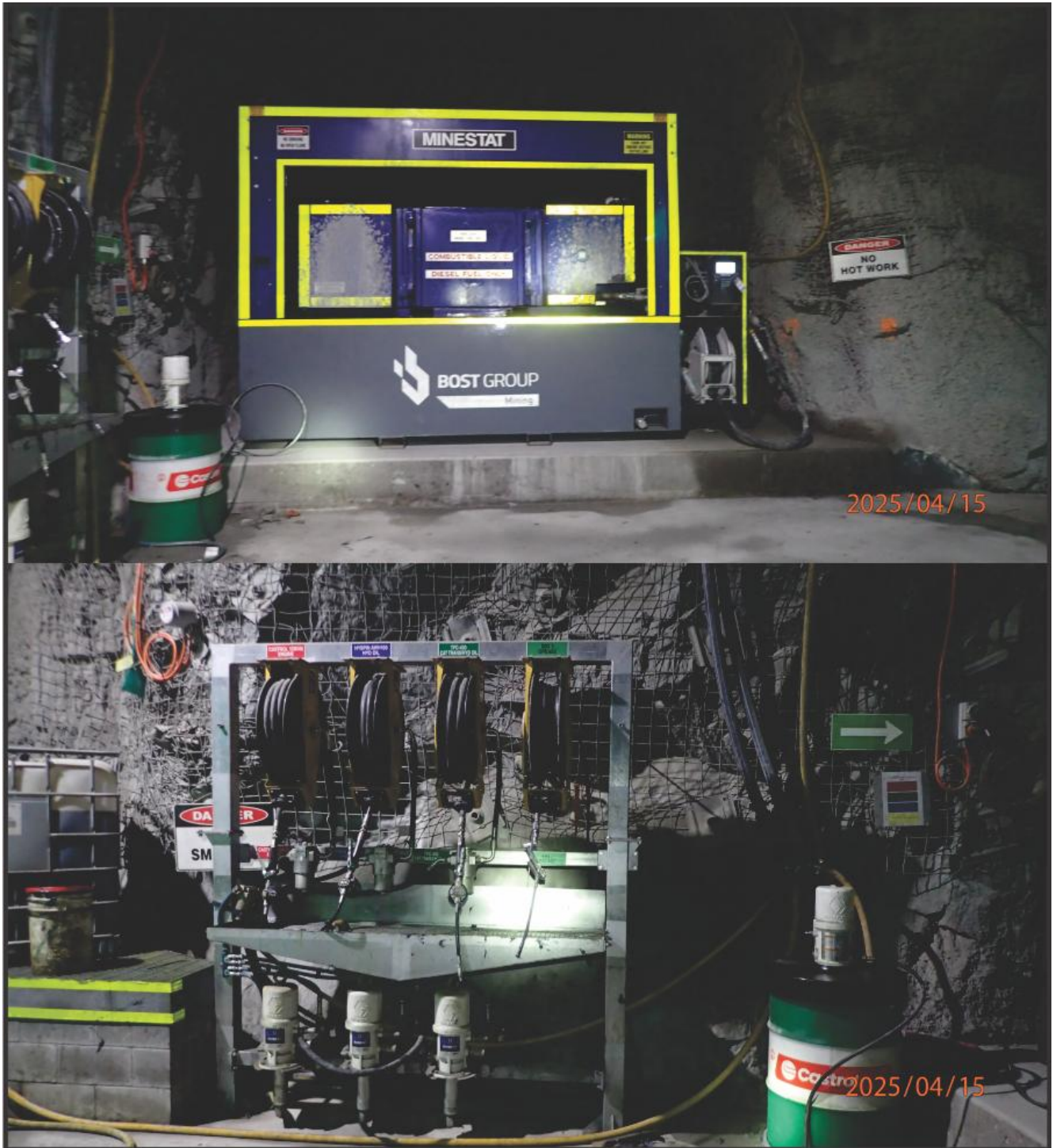
Figure 18-3: Roswell refuelling and lubrication facilities
