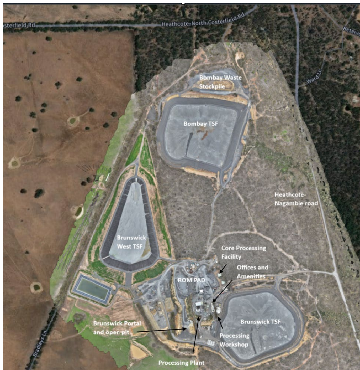
Figure 14: Brunswick Site, including processing plant, offices, exploration facilities, and tailing storage facilities
