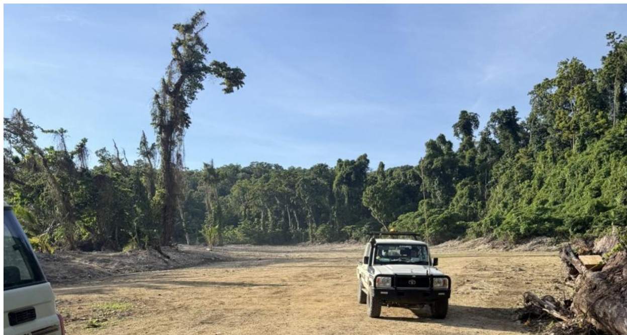
Project enabling works – clearing at the wharf and DSTP site completed during the reporting period
