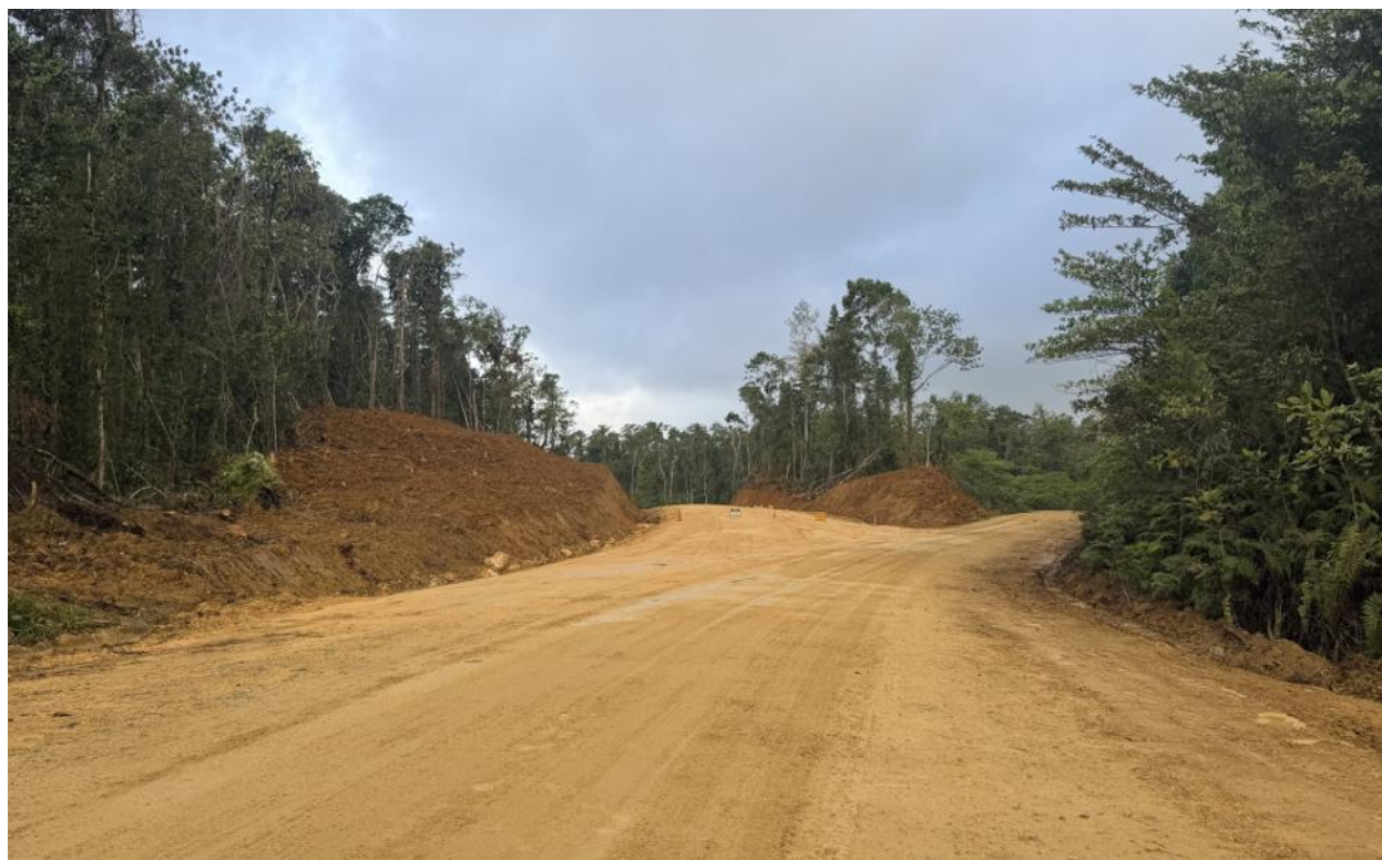
Woodlark Island - road upgrades well underway
