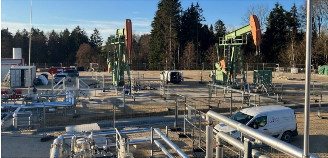
Figure 10: Photograph showing the Anshof-3 well (left side, photo) and the Anshof-2A well (right side, photo) producing into the PPF
