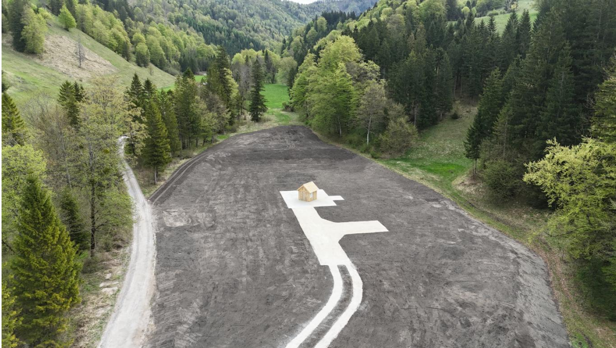
Figure 24: Photo of Welchau-1 drilling site area after partial recultivation
