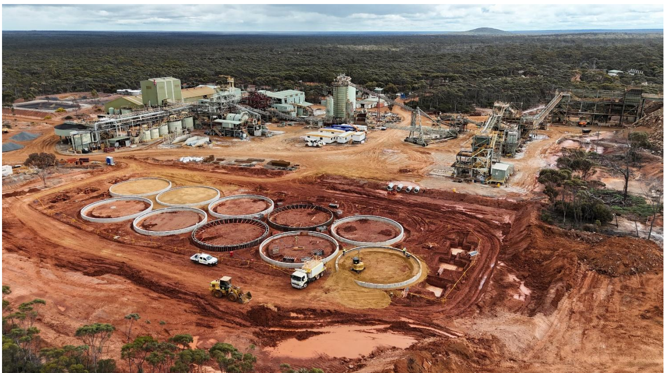
Image 3: CIL Tank construction - Lake Johnston Processing Facility
