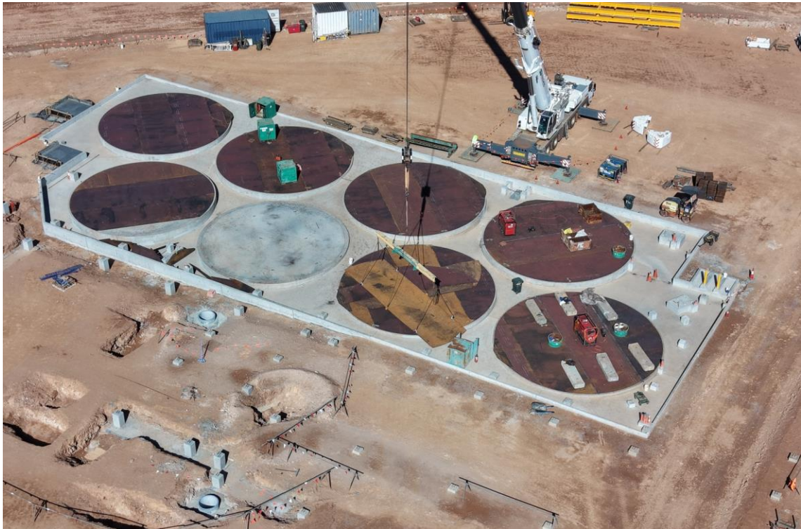
Figure 4: CIL circuit – major concrete works complete, tank construction commenced
