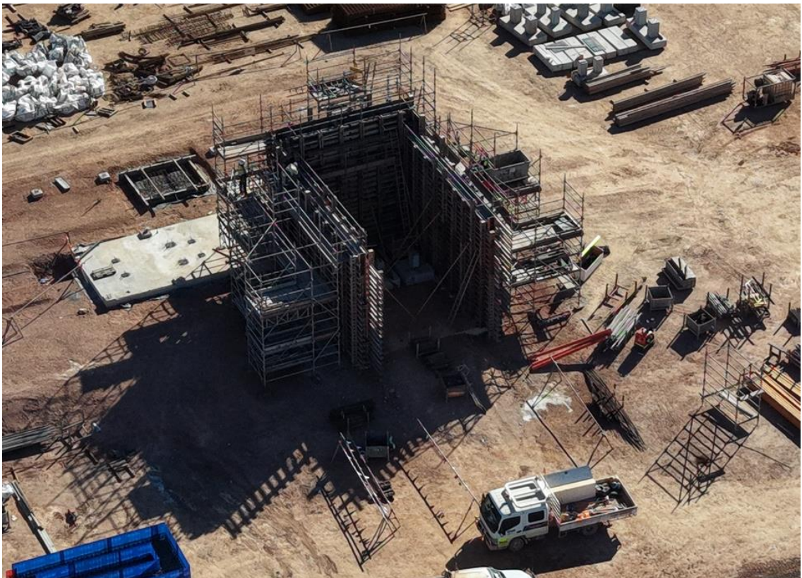
Figure 5: Surge bin and wall foundations
