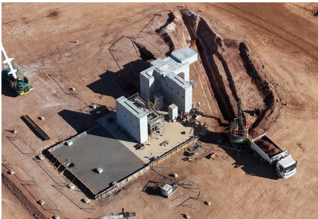
Figure 3: Grinding and Classification area – major concrete foundations complete
