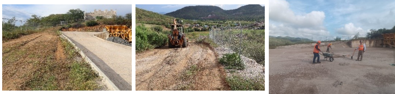
Figure 5: Rehabilitation of the access road to the Plant and preparation of the crushing yard
