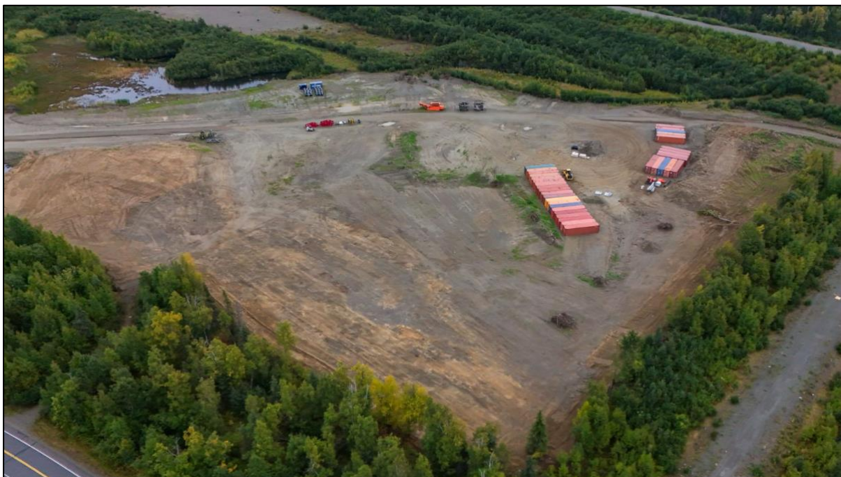
Figure 4. Aerial view of Nova Minerals antimony processing plant site which has been prepared ready for construction
