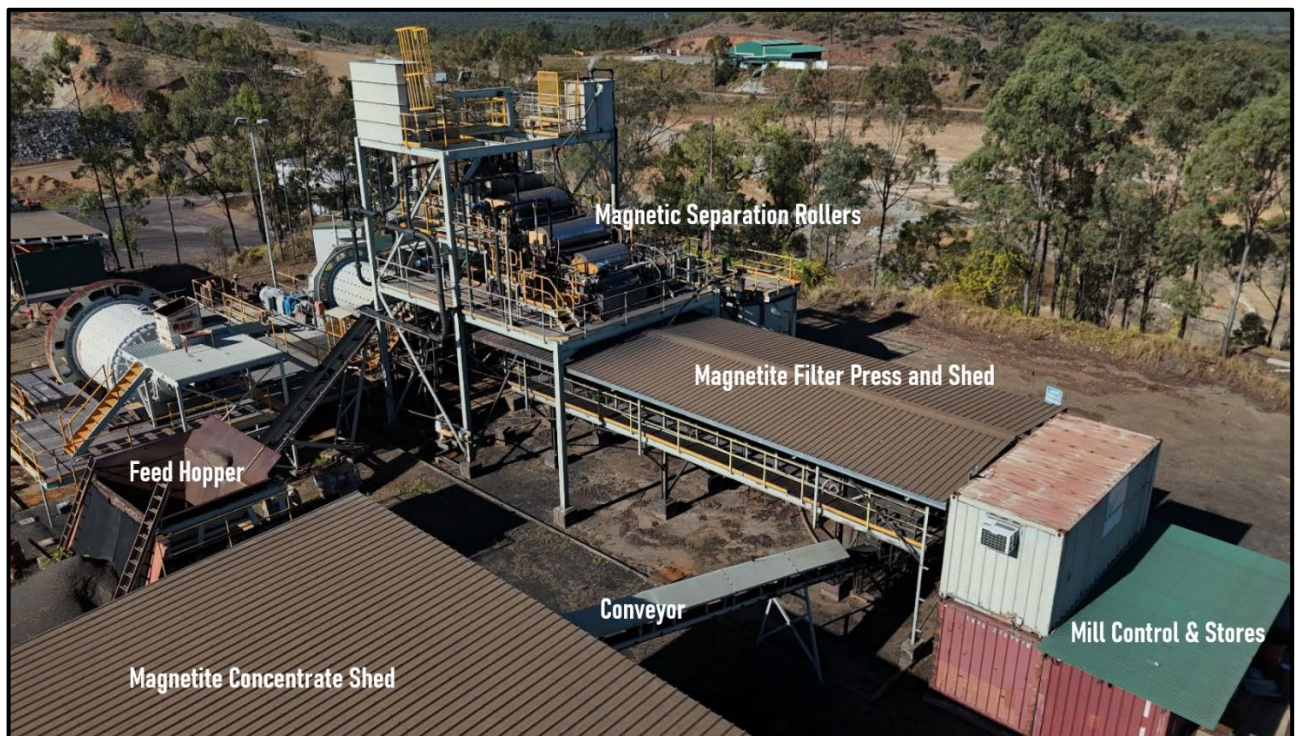
Figure 2: Mt Moss Mill with all magnetite-related plant on July 13, 2026.
