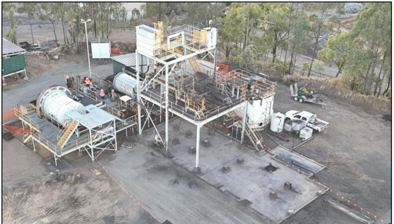
Figure 3: Mt Moss Mill with all magnetite-related plant decommissioned on August 10, 2026. Ball mills have since been emptied, with liners stripped and lifted.
