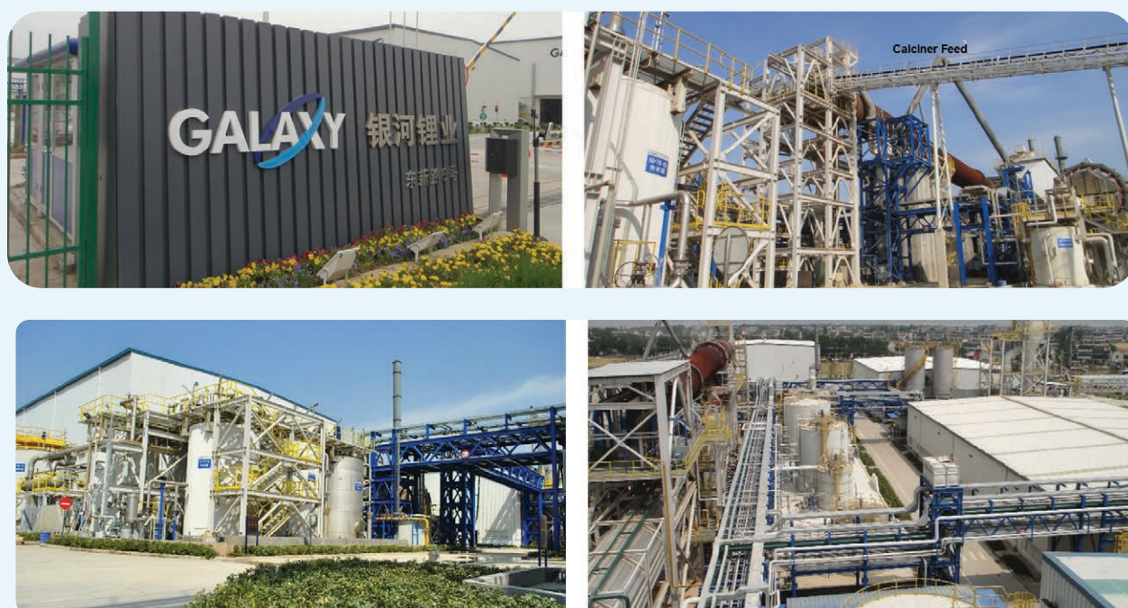
Figure 10: Galaxy Jiangsu Lithium Carbonate Plant
