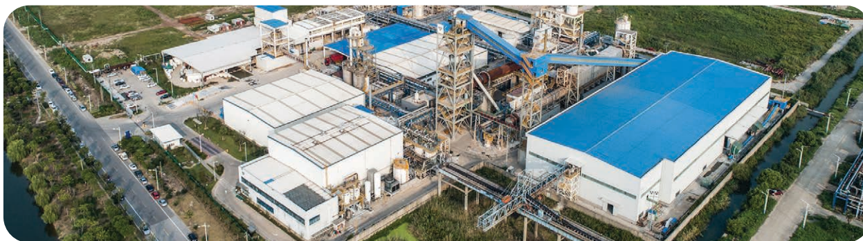
Photo: Galaxy's Jiangsu Lithium Carbonate Refinery, Jiangsu Province, China
