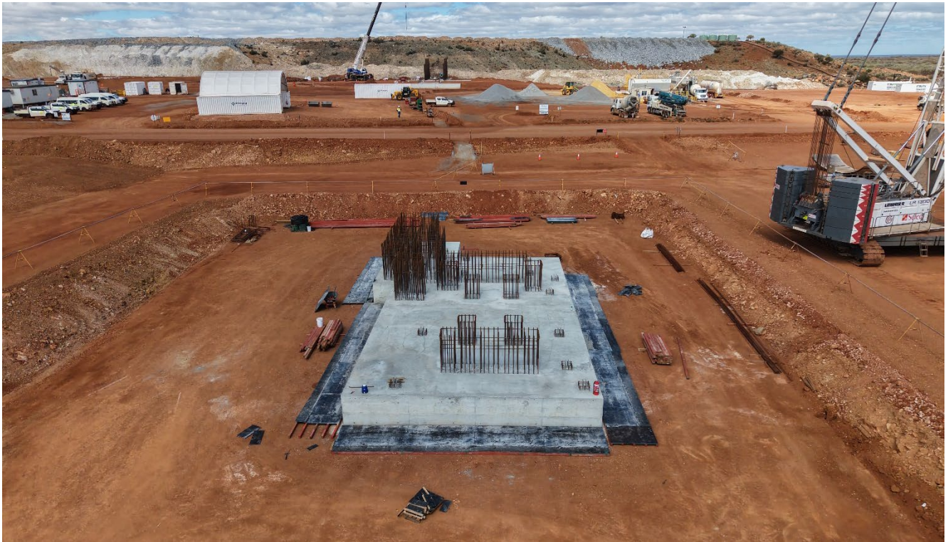
Figure 4 – Ball mill foundation poured
