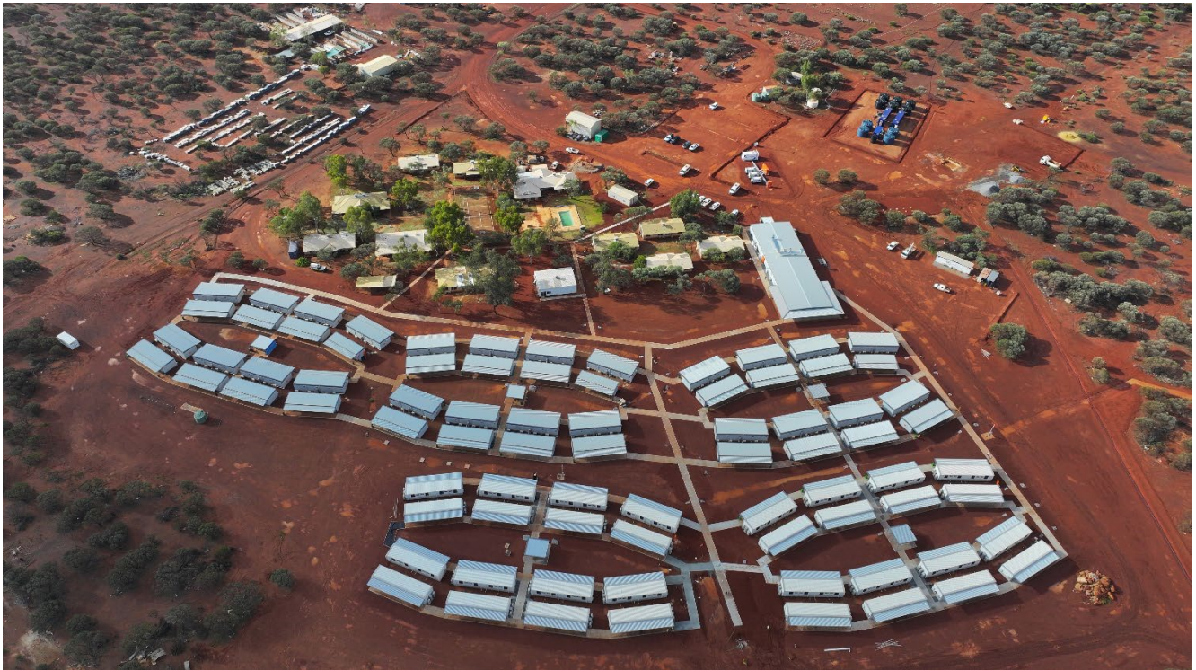
Figure 10 – Youanmi 351 room camp facility
