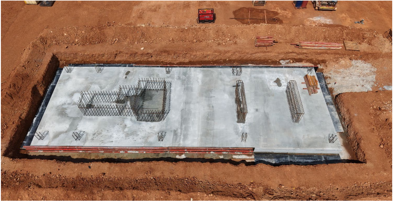
Figure 5 – ISAMill foundation poured
