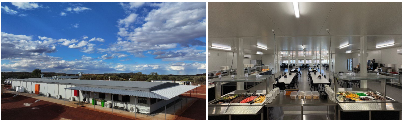
Figure 11 – Youanmi dry mess facility operational
