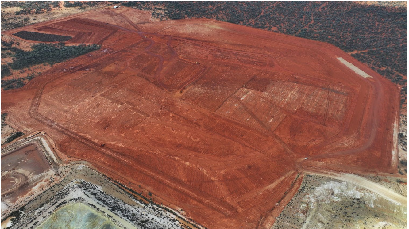
Figure 8 – Tailings Storage facility
