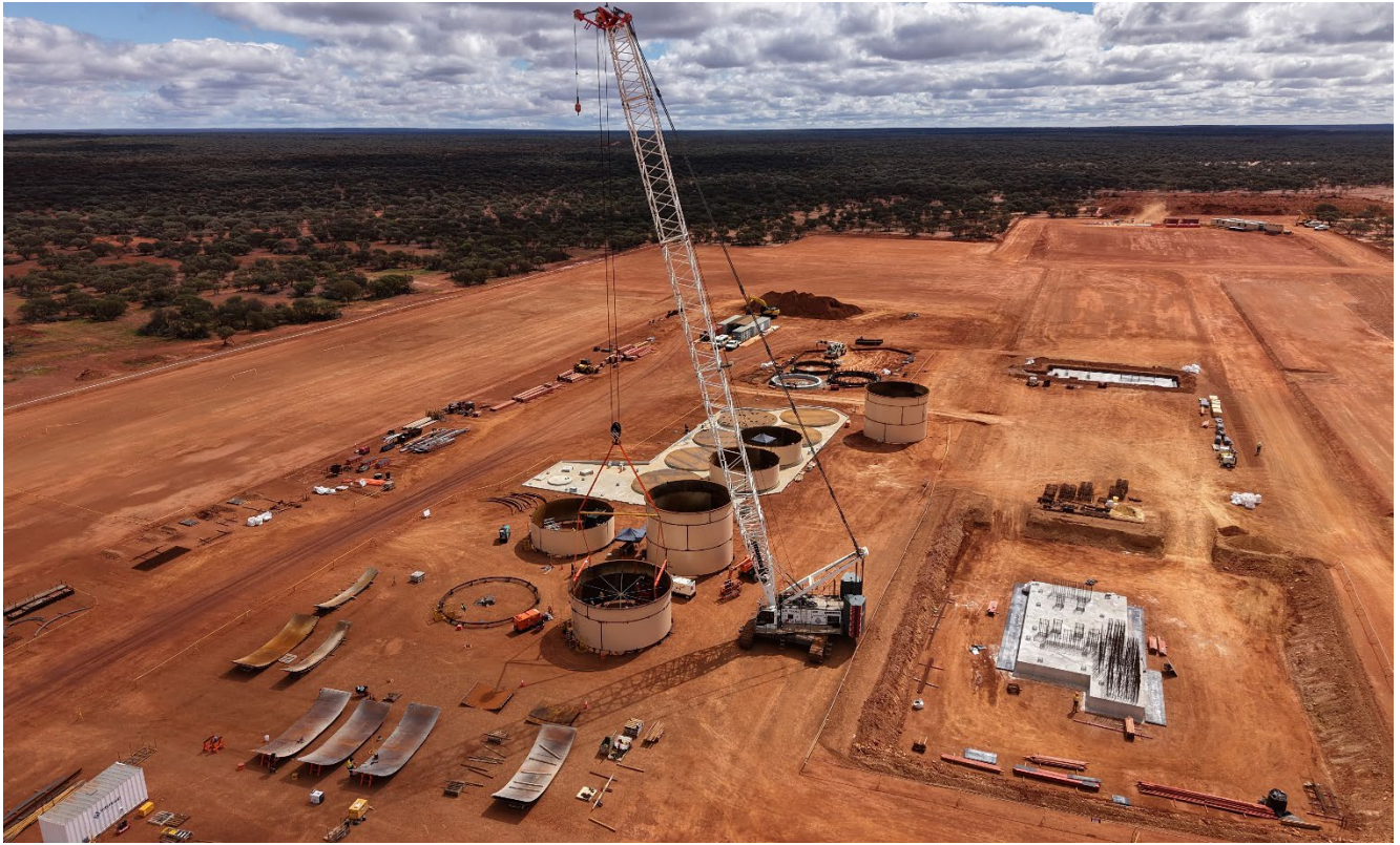
Figure 1 – Progress of construction on site – looking South
