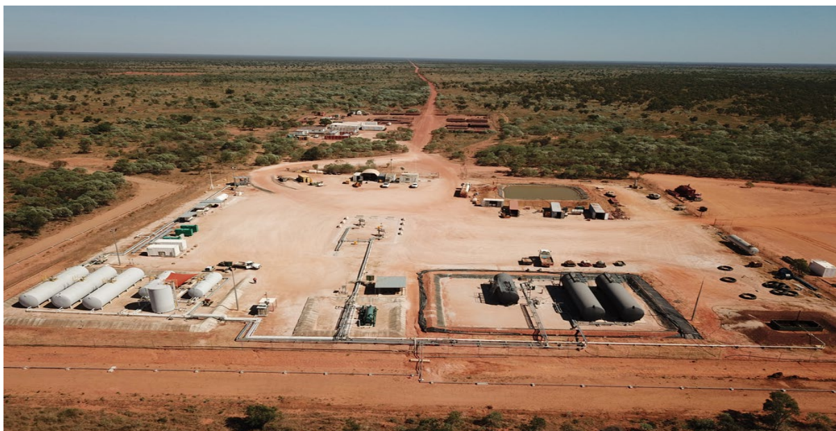
Figure 7 – Ungani Production Facility
