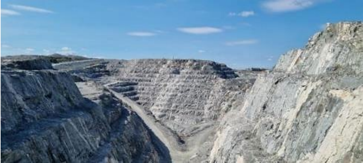
Figure 2-1: View of the Phase 1 Open Pit Operations
