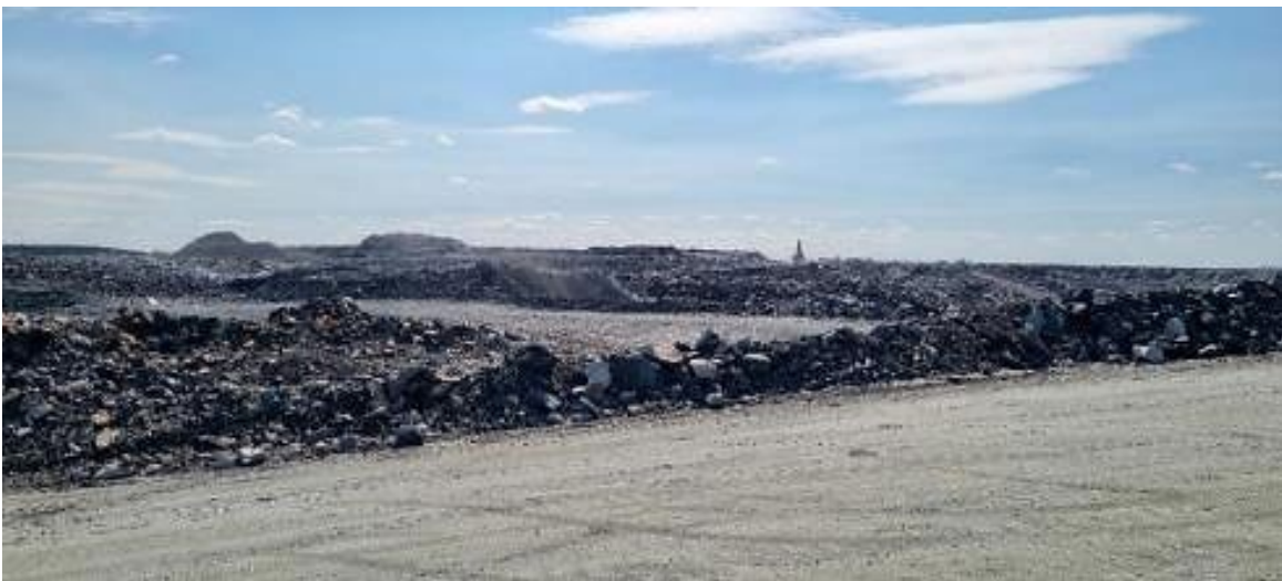
Figure 2-3: View of the Phase 3 Open Pit Operations
