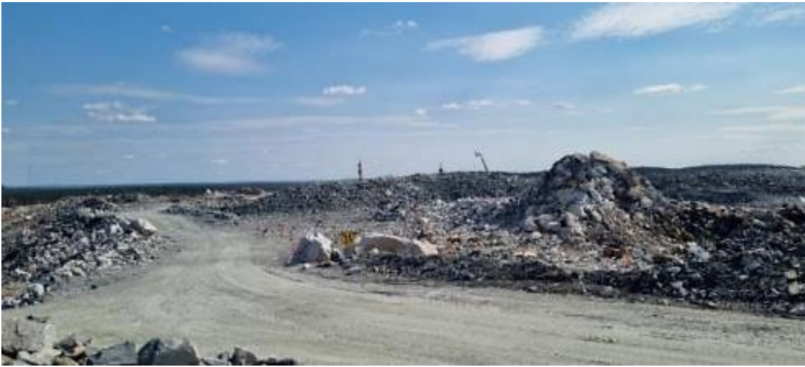
Figure 2-2: View of the Phase 2 Open Pit Operations
