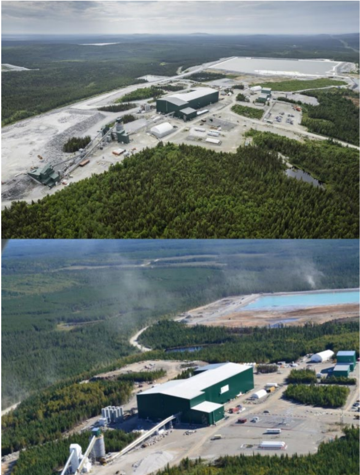
Figure 5-3: View Looking South-Easterly Showing the Plant Facilities in the Foreground of the Tailings Impoundment Area
